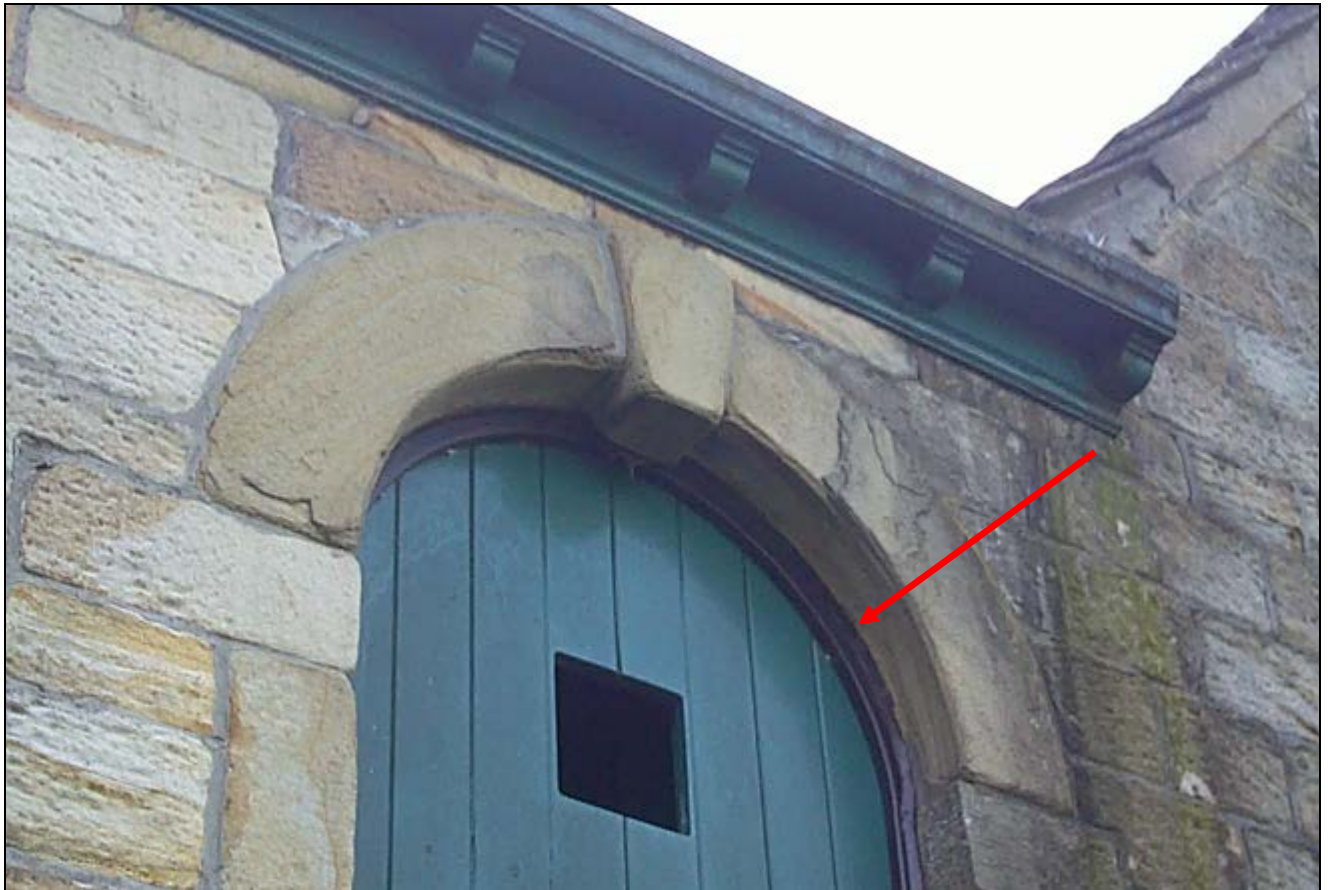
Detail of hayloft shutter on front elevation, showing framing (indicated) still in situ of the probably 1980s glazing it replaced
