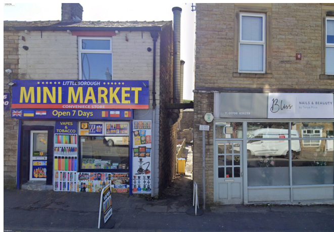
View from Church Street towards the site
