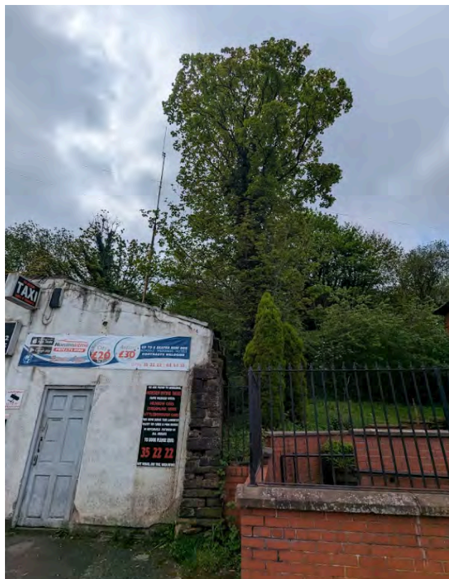
Photographic plate showing the stone retaining wall and the difference in ground level between the plot and T1. (ROAVR, 2024)
