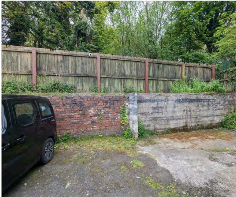
Photographic plate showing the masonry retaining wall and the difference in ground level between the plot and T4, T5 and W1 in the background of the image. (ROAVR, 2024)
