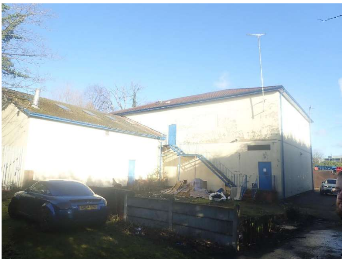
Photograph 2 – The south-eastern and south-western aspects of the building.
