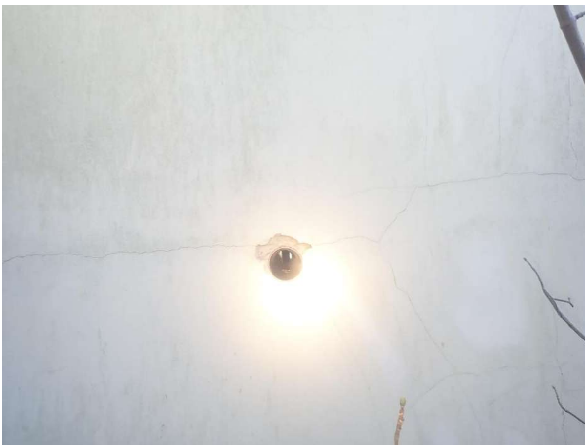
Photograph 6 – Vent hole on the north-western aspect of the building.
