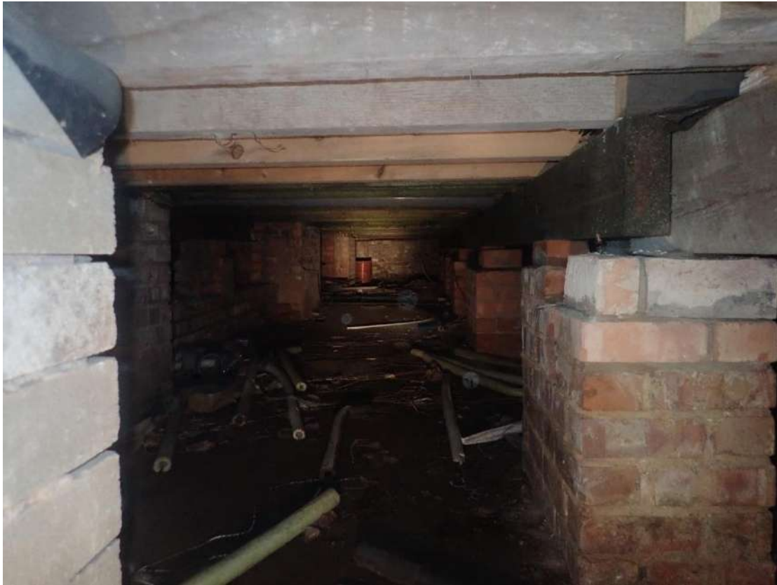
Photograph 13 – The crawl space under the building.
