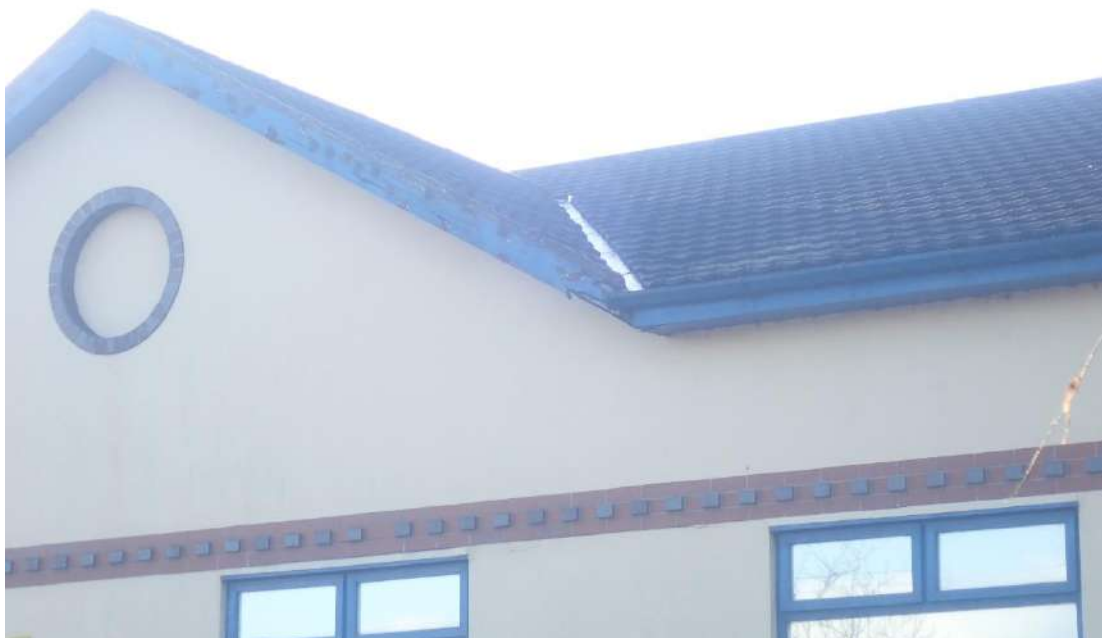
Photograph 3 – The gable on the north-eastern aspect of the building, showing the damaged boxed soffit.
