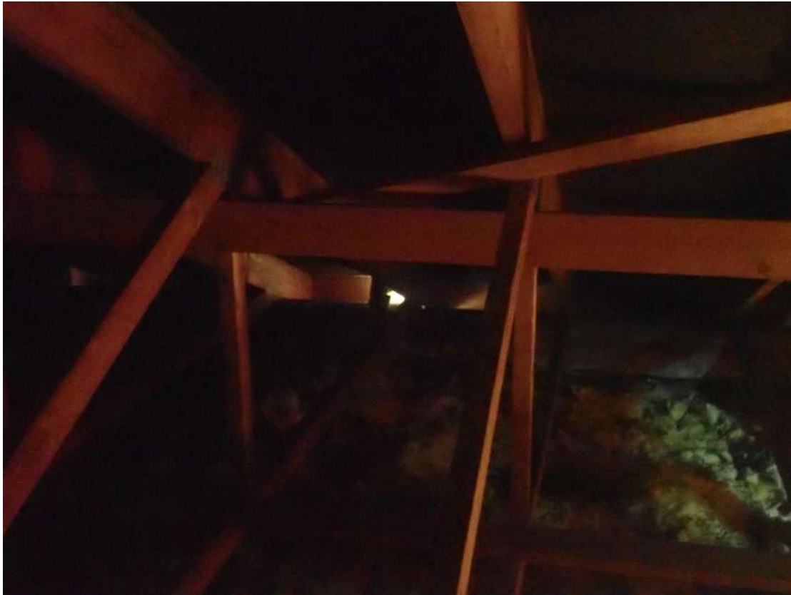
Photograph 9 – Light ingress from the eaves in the loft void.
