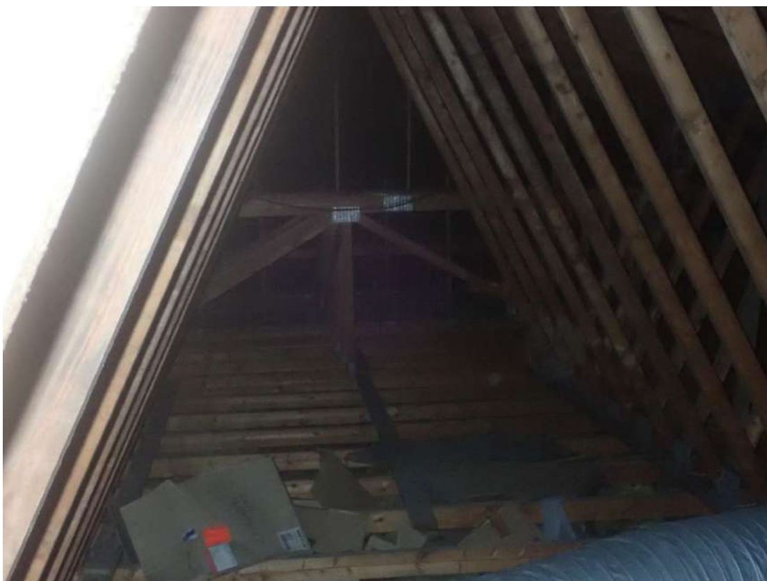
Photograph 7 – Centre of the loft void.
