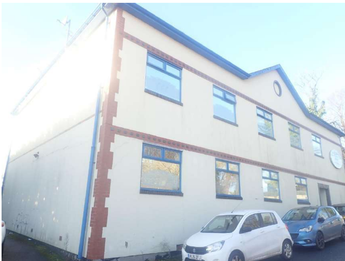
Photograph 1 – The south-eastern and north-eastern aspects of the building.
