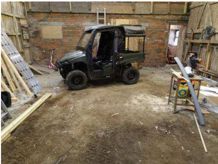
Photo 2. Exposed soil ground to barn interior with stone flags in background.
