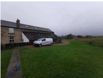
Photo 9. Rear NE side garden and elevation.
