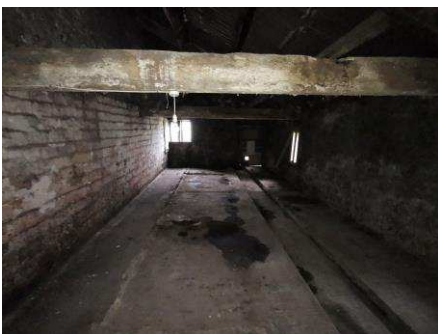
Photo 4. Concrete floor slab to shippen.
