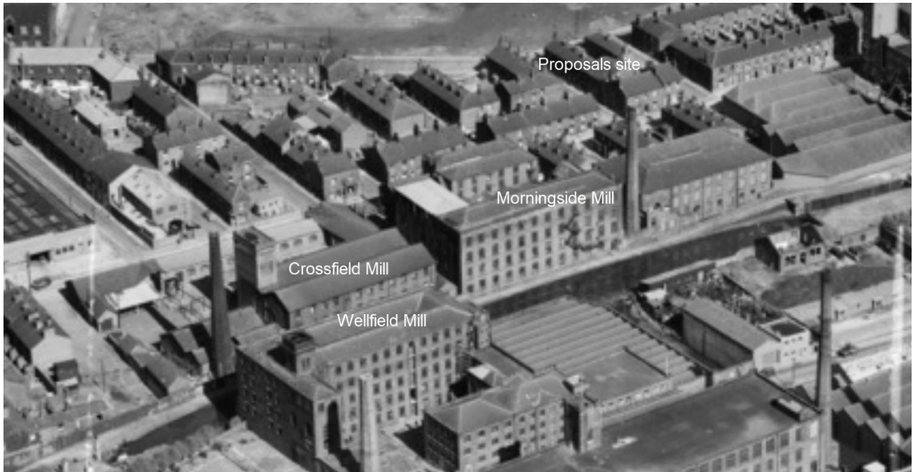
Figure 9) Aerial view (1953) showing Crossfield and adjacent mills and terraced housing on the proposal site to the north
