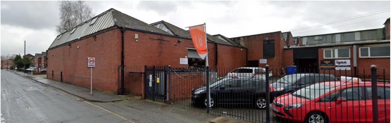
Figure 7) Northlight roof weaving sheds south of the site
