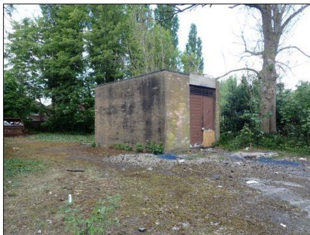
Photo 10: Building 2, eastern and southern elevations
