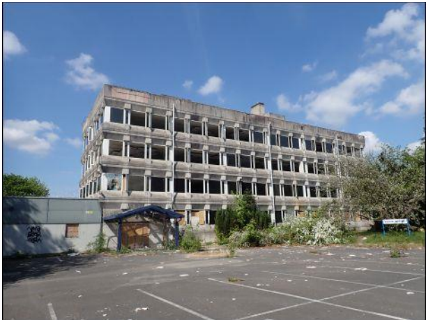
Photo 6: Building 1, eastern elevation
