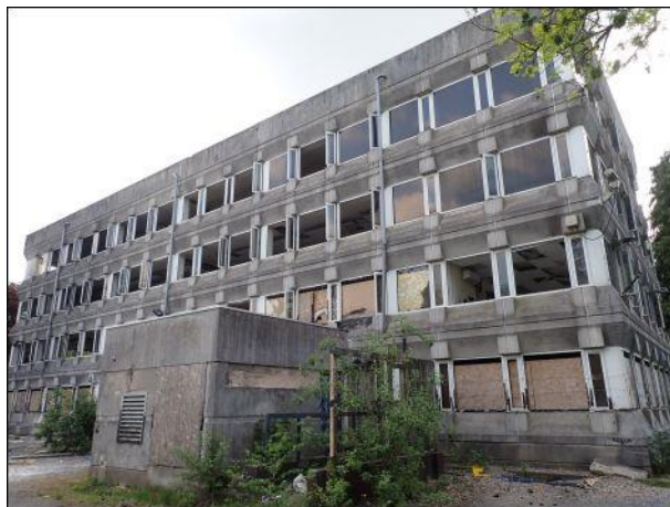
Photo 8: Building 1, north-western corner
