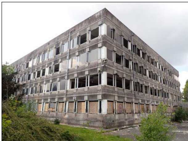
Photo 7: Building 1, north-eastern corner
