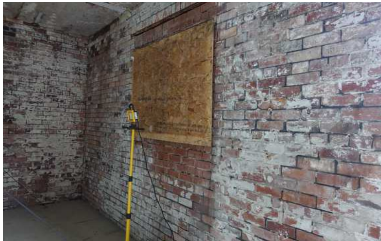
Timber boarding to interior of duct present within bricked up window.
