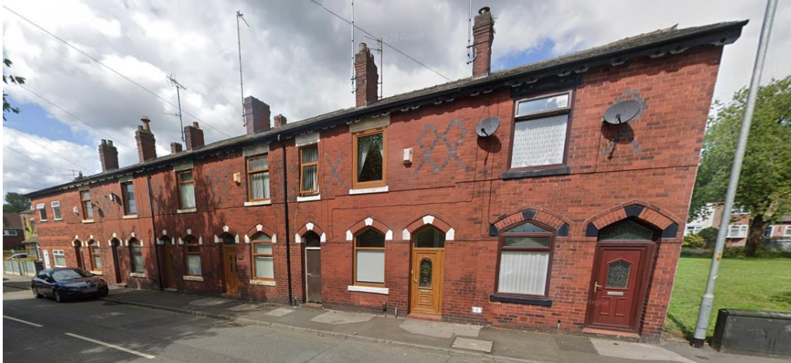
Photo. 2 Existing terrace along Boarshaw Road
