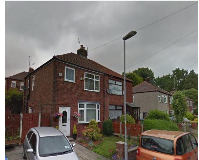
Photo. 3 Existing semi detached housing to Brassey Street (rear of site)
