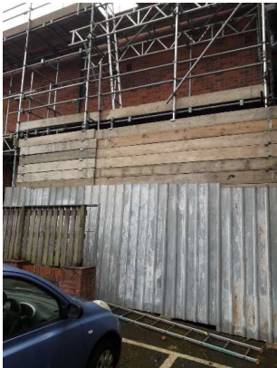
Additional hoarding – scaffold on-going
