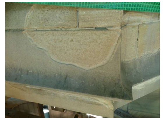
Loose/spalling stone removed and face cut back to shed water. Edge contrast to be softened using a conservative DOFF cleaning
