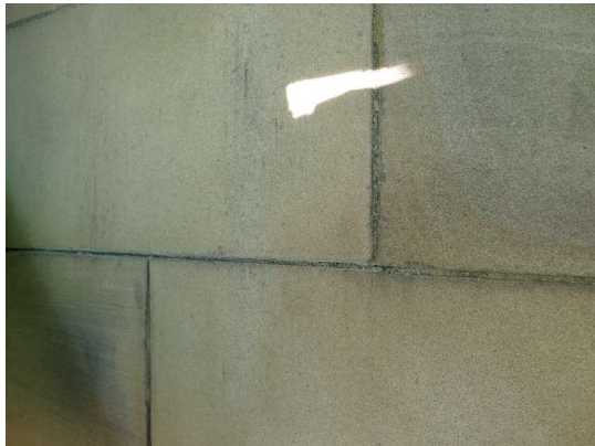
Joints cut out to the facing stonework
