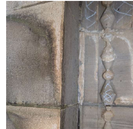
Loose/spalling stone removed and face cut back to shed water. Edge contrast to be softened using a conservative DOFF cleaning
