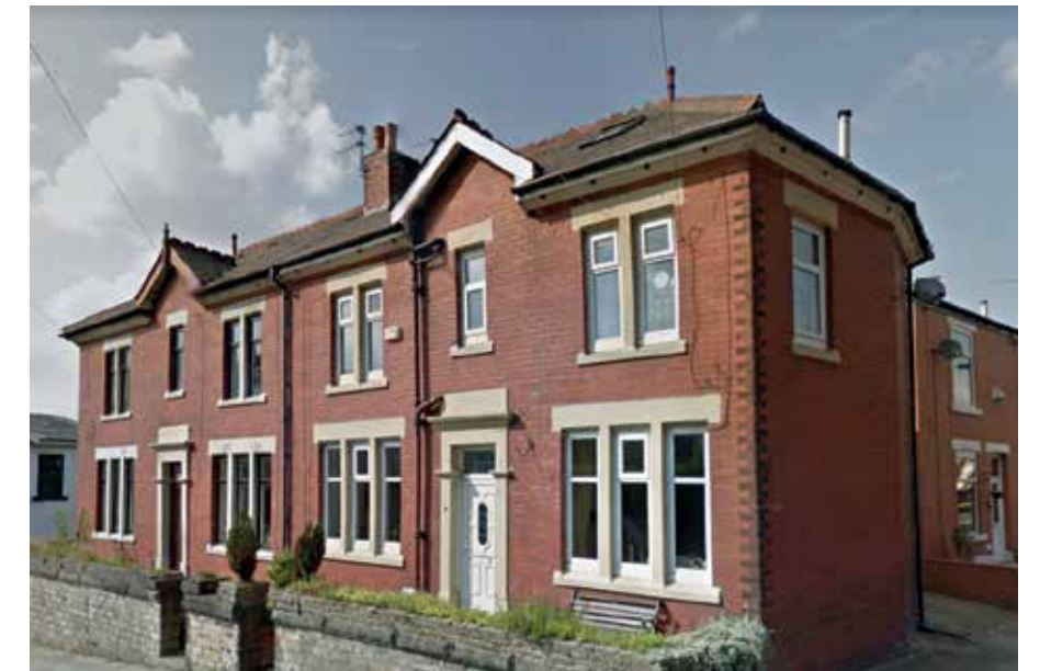
Pair of large semi-detached houses on Vicarage Road North with corbal detailing, finials and stone mullion windows.
