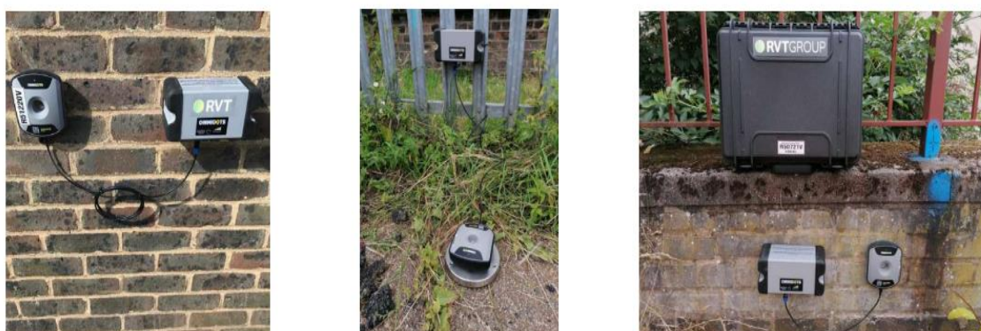
Figure 5.1 - vibration monitoring equipment
