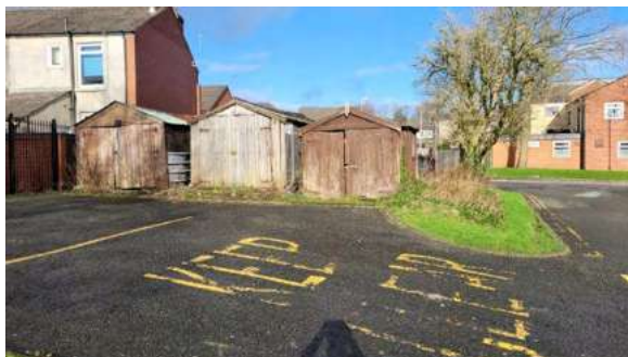
Block B – Existing Garages from the South
