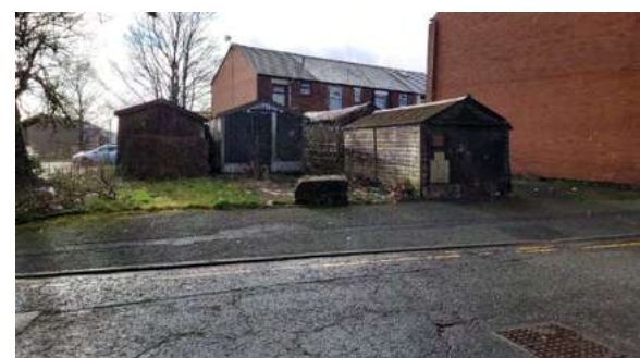
Block B – Existing Garages from the North
