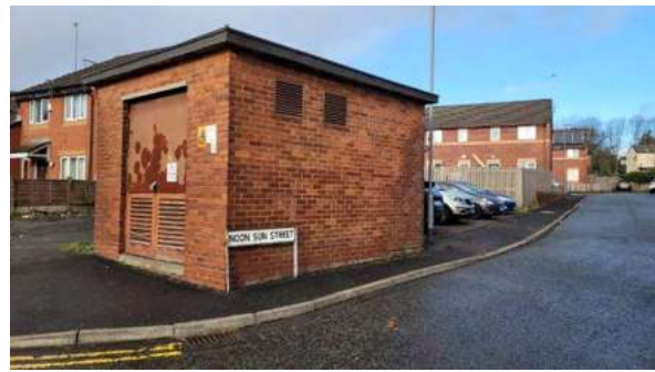
Block C – Sub Station with Site Beyond
