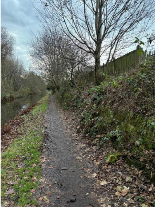
Photograph 5: The canal tow path, a retaining wall, slope and secure wooden fence along the top of the slope separates the canal from the proposal site. Very limited ecological connectivity for riparian mammals.
