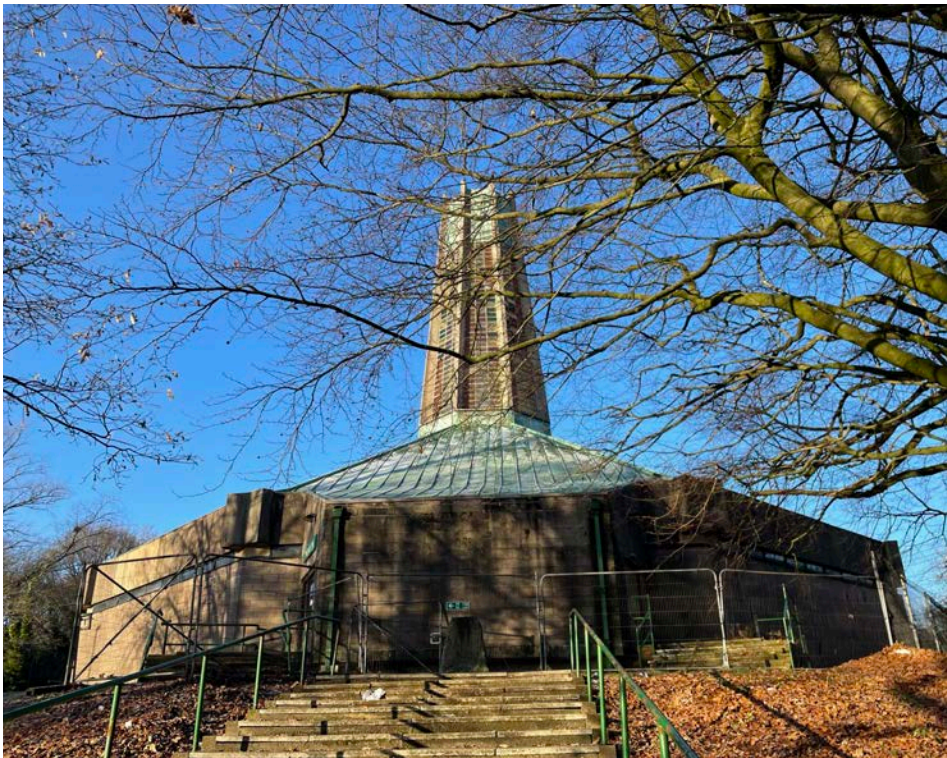
9 View from the existing stepped access up the hill towards the building from the South-
