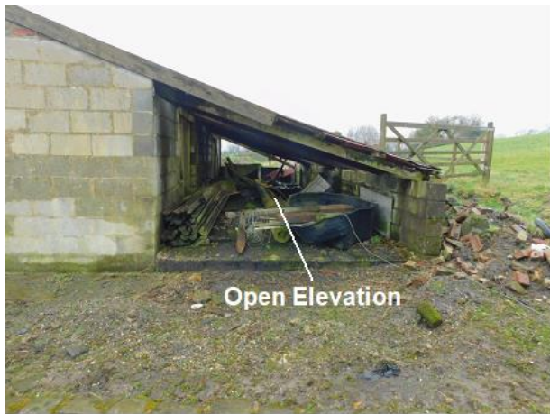
PHOTO 1 North-eastern Corner of Lean-to
