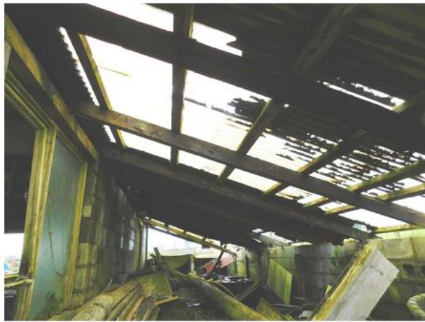
PHOTO 15 Underside of Lean-to Roof
