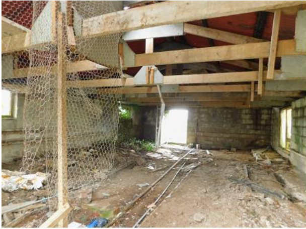
PHOTO 13 View Within Main Building
