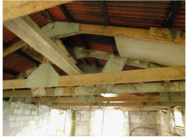
PHOTO 14 Underside of Main Building Roof
