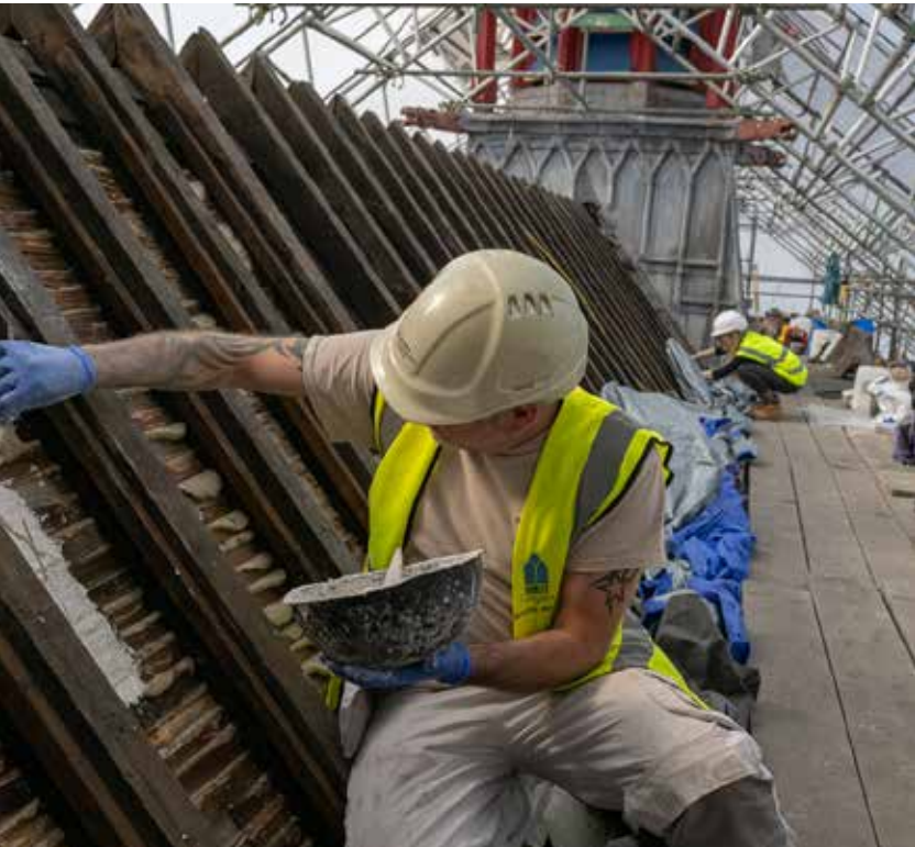
4.3 Panels Being Consolidated
