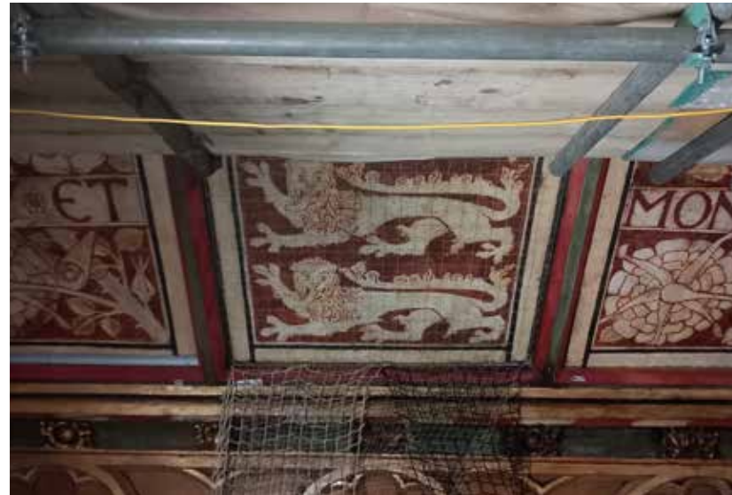
4.6 Test Panel Installed
