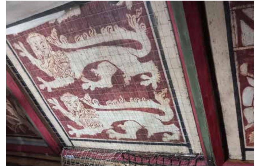
4.7 Test Panel Installed
