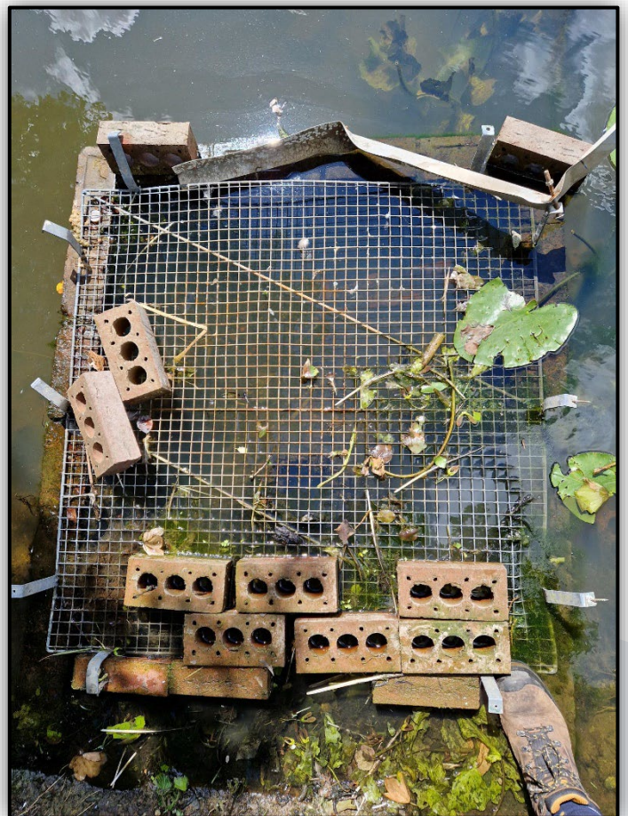
Fishery Lake Outfall Chamber & Pipe View
