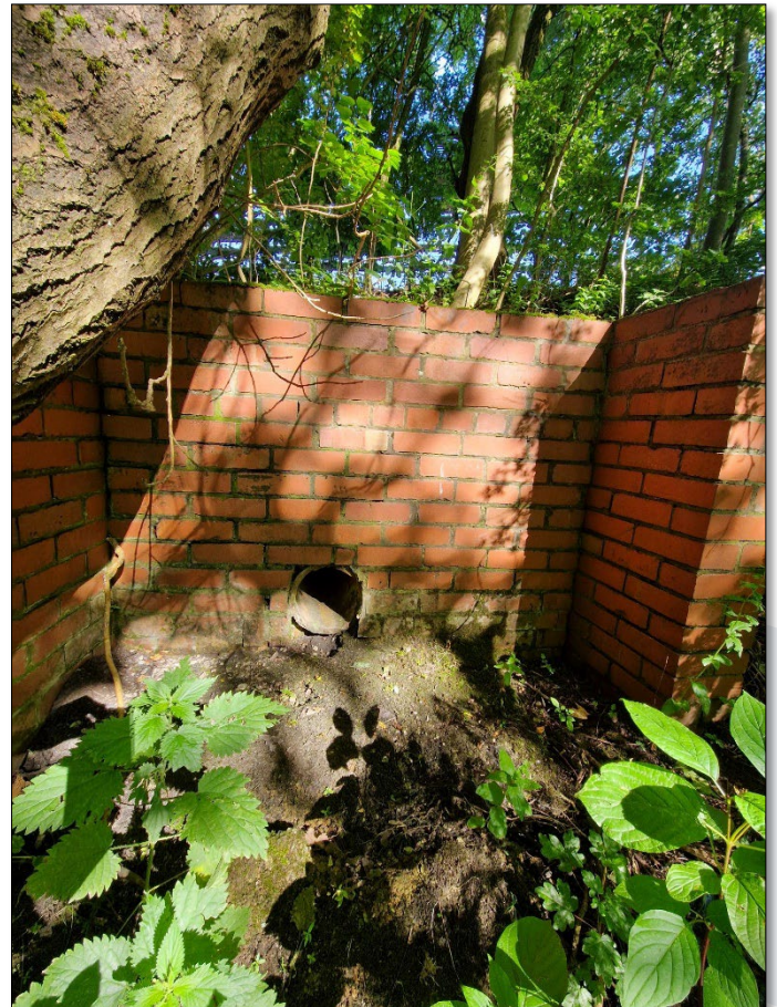
Pond Inlet Headwall
