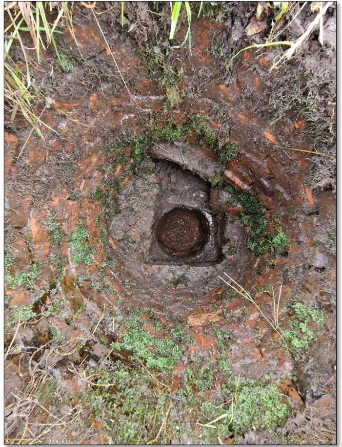
MH3 Internal View
