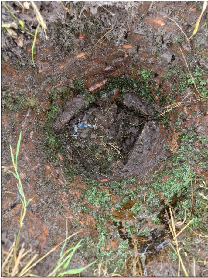
MH3 Internal View During Clearing
