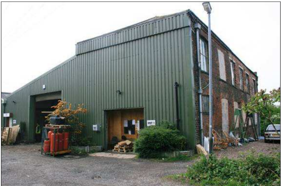
6. View from northeast showing the brick principal elevation of the building and clad northeast elevation
