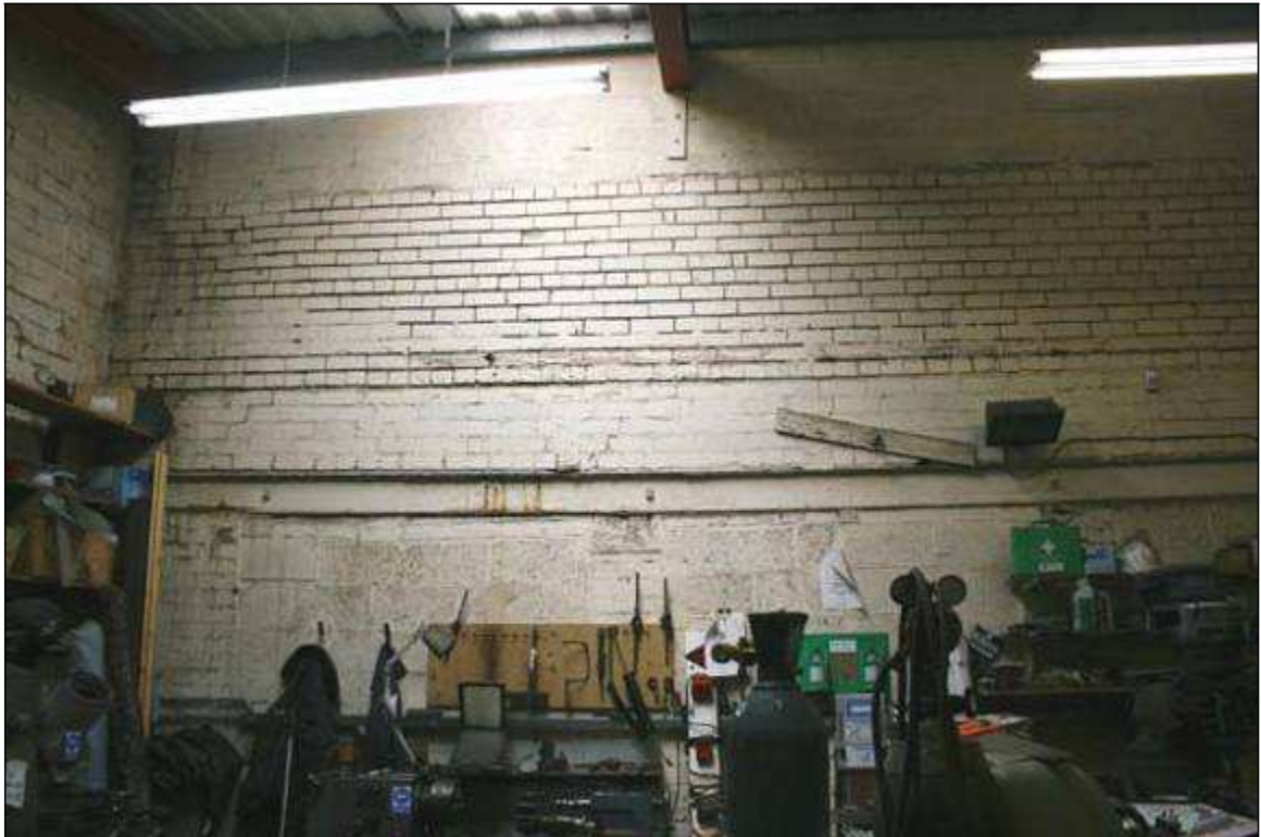
22. Rear wall of rear wing of principal building showing blocked opening to outshut
