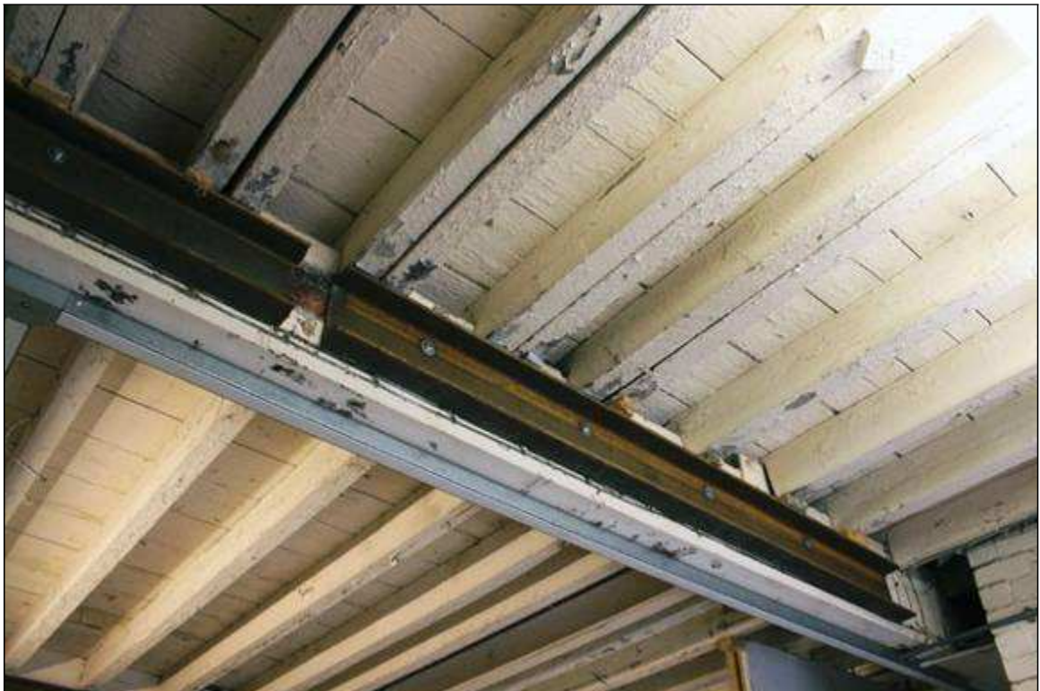
21. Detail of ceiling construction, with heavy beams and closely-spaced joists
