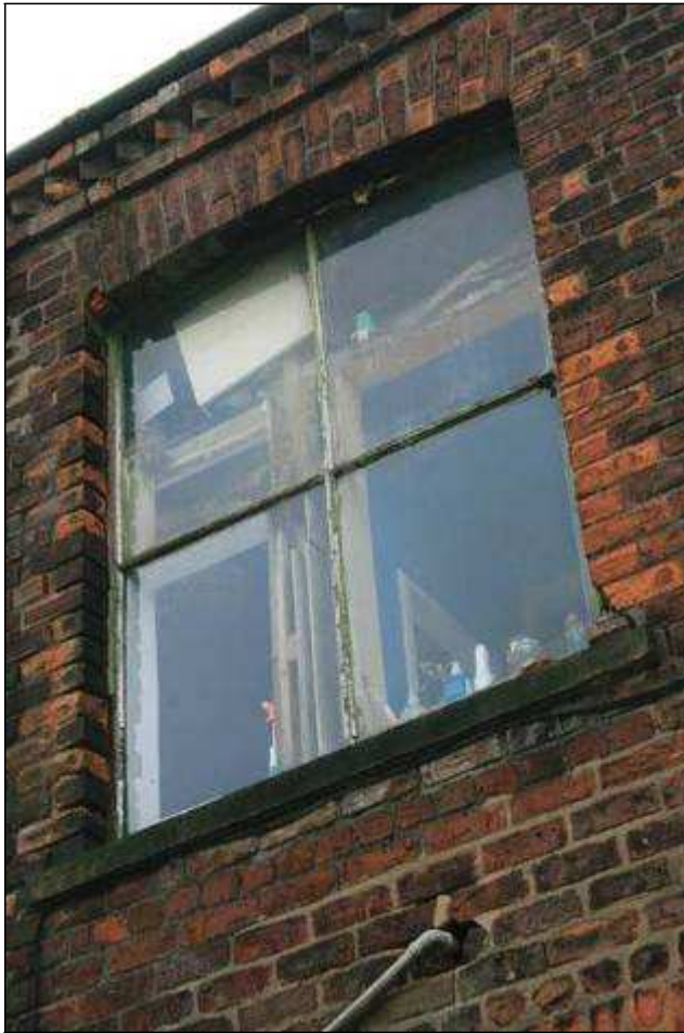
15. Four-pane, probably original, glazing of first floor window in first bay; also dogtooth eaves cornice
