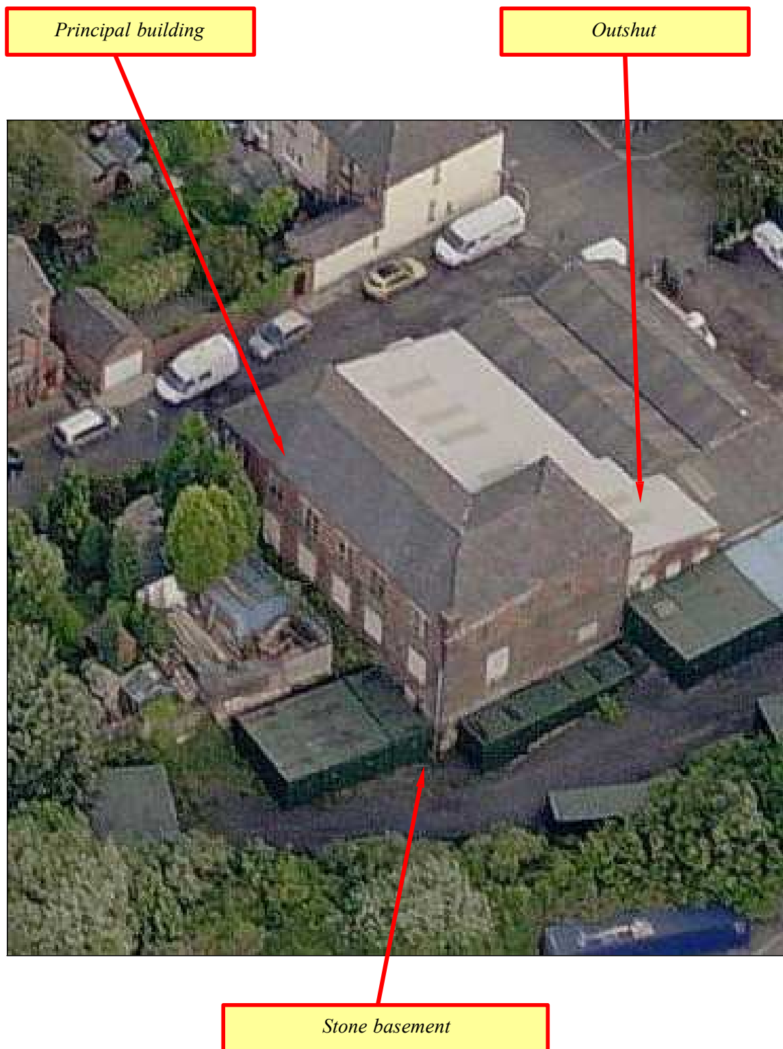
7. Elements of the building (based on GMAU photograph)
