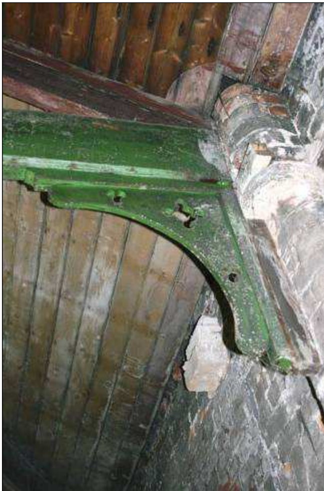
24. Boarded arch applied to roof truss forming hip at southwest end of main range, suggesting a dais or proscenium
