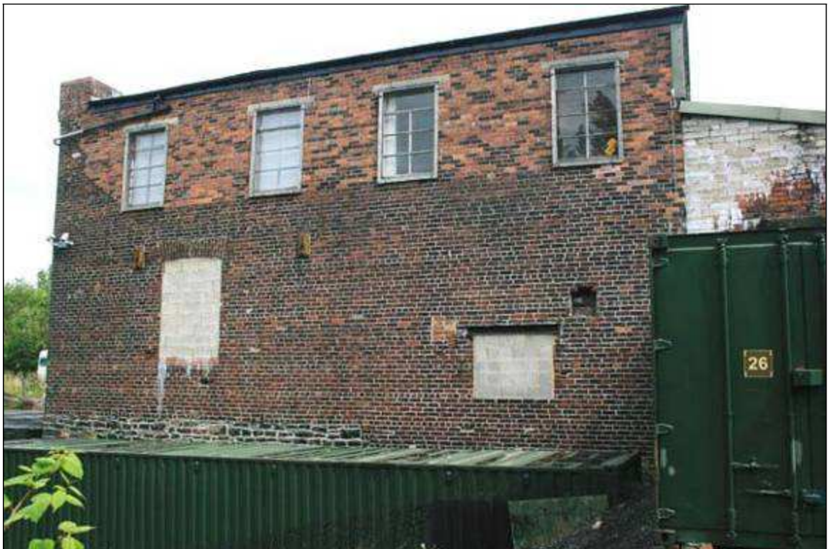
16. Southwest elevation, showing first floor rebuilding
