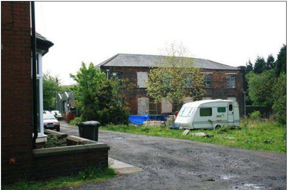
1. Setting: looking south from the northern end of Brown Street to the building
