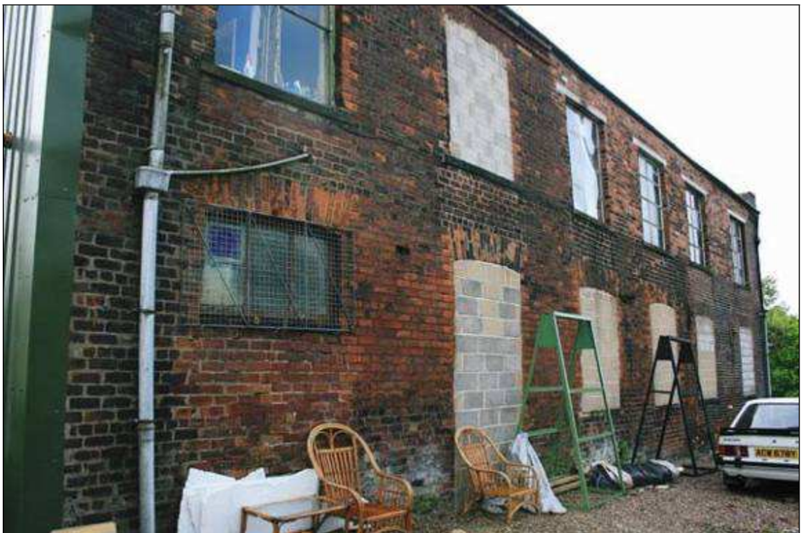
12. Closer view showing blocked windows
