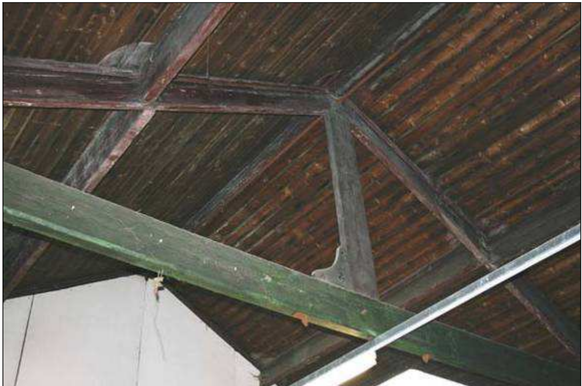
8. Roof truss with small surviving brace to kingpost
