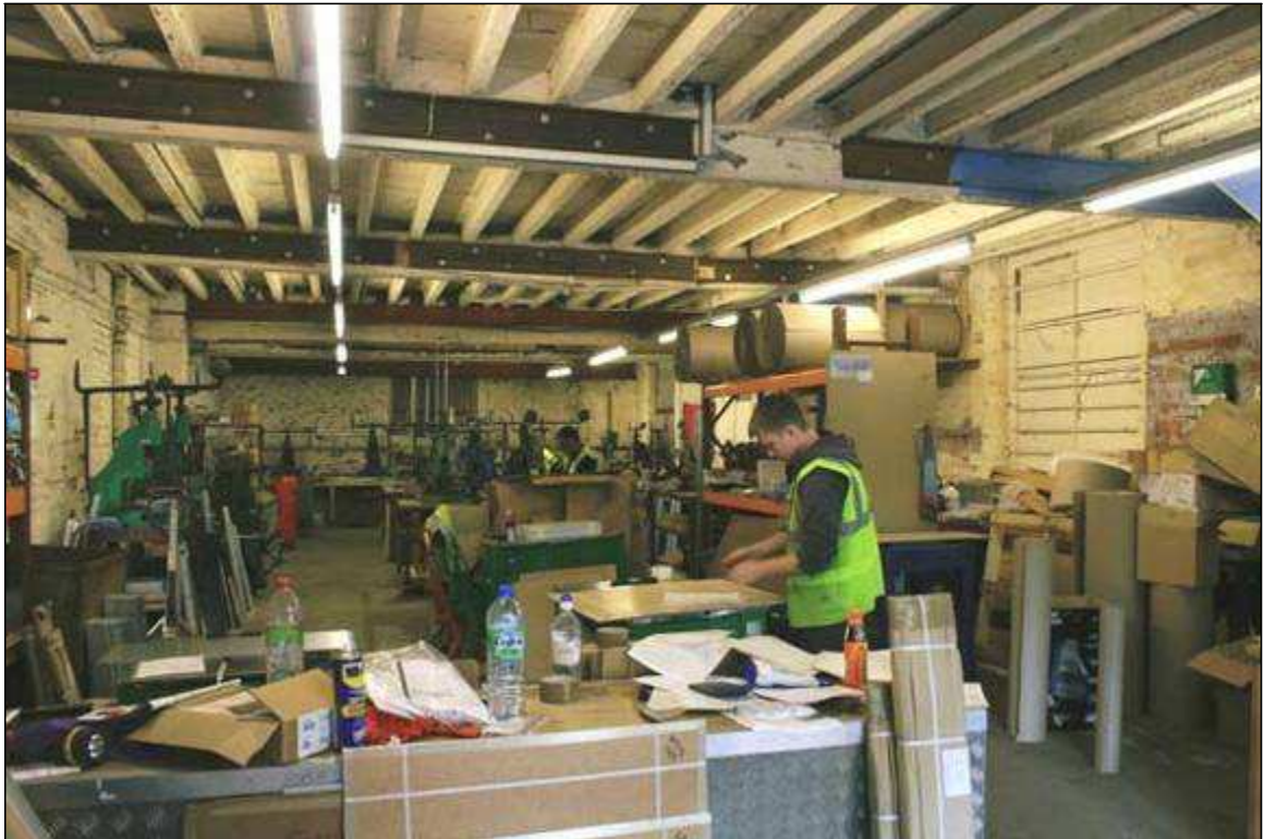
20. General view of ground floor of main range, looking southwest
