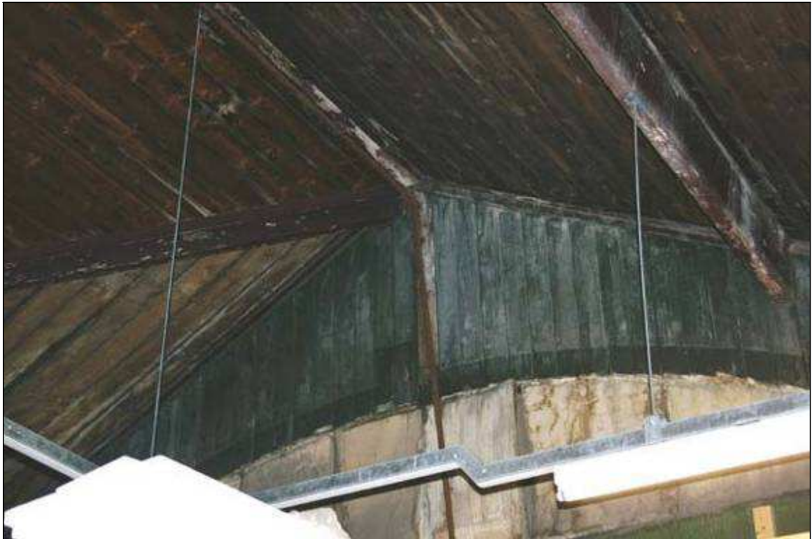
24. Boarded arch applied to roof truss forming hip at southwest end of main range, suggesting a dais or proscenium
