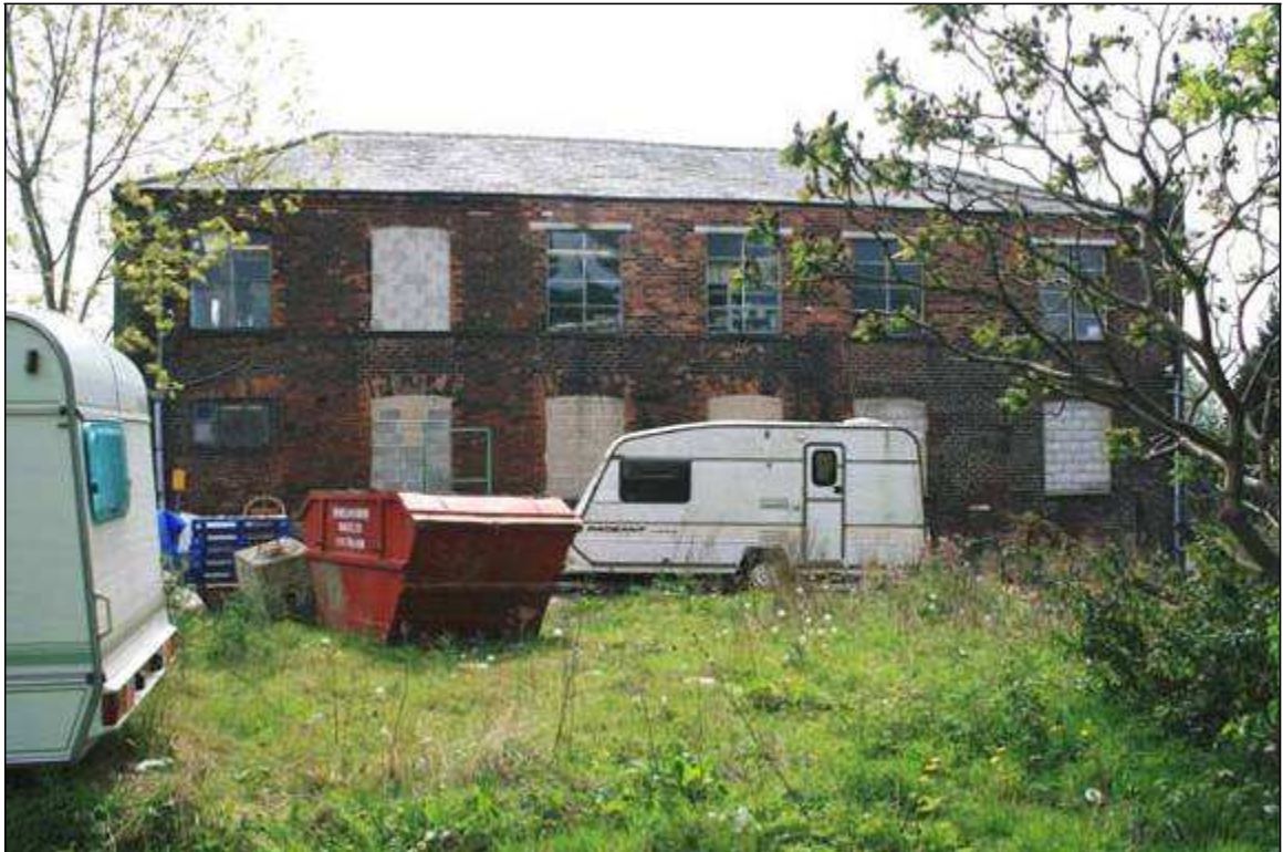
11. Main elevation of principal building, from northwest
