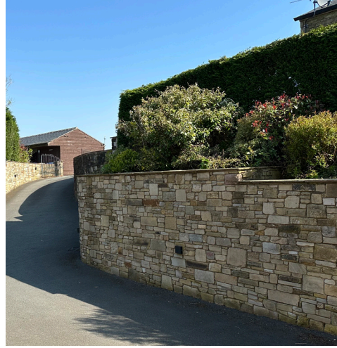
2. Existing Wall Retained
