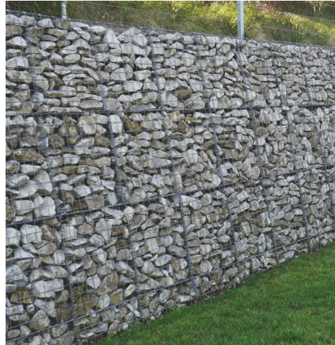
6. Gabion Retaining Wall
