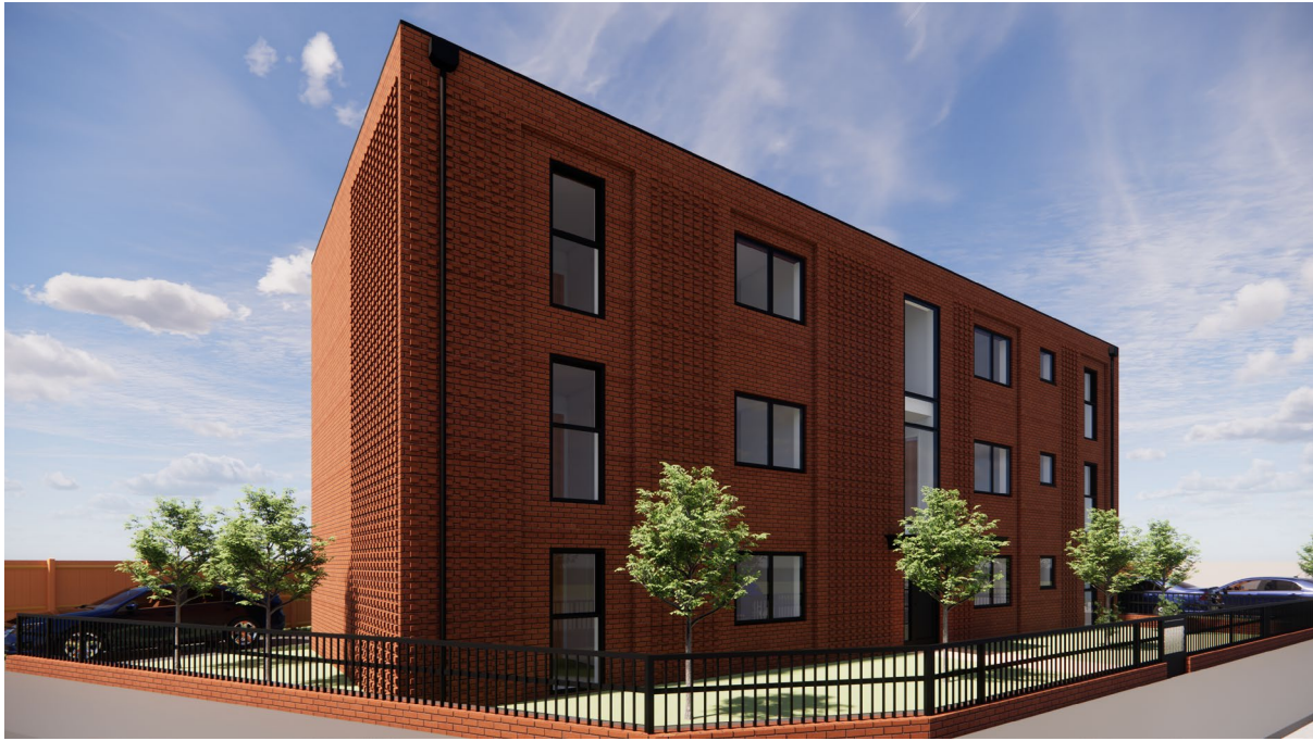
Fig 16: Street View showing Brick teething feature on proposed development.
