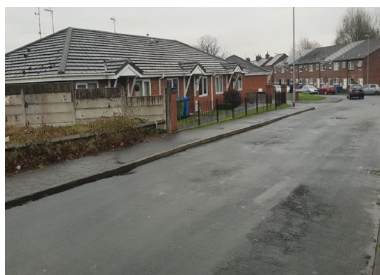
Fig 10: Bungalows along Joseph Street.
