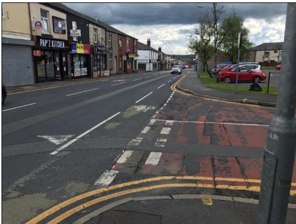
Figure 2. A671 Whitworth Road in vicinity of site
