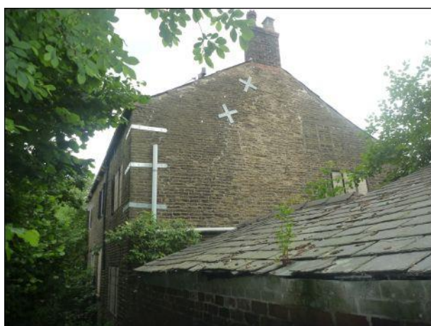
Photo 23: Building 3, south-eastern and south-western elevations
