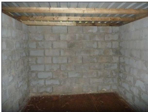
Photo 37: Building 4, section 4.4 internal area
