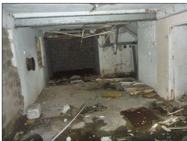
Photo 35: Building 4, Section 4.3 internal area
