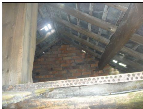
Photo 36: Building 4, section 4.3 roof void
