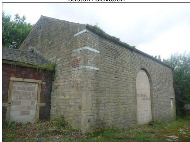
Photo 17: Building 2, south-eastern gable end and north-eastern elevation
