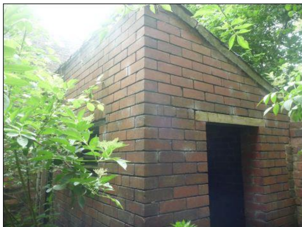
Photo 19: Building 2, single-storey extension
