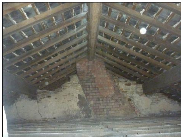
Photo 26: Building 3, roof void at north-western end of the building
