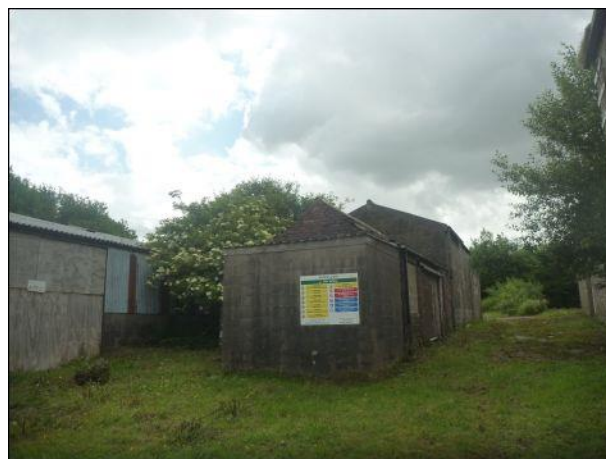
Photo 30: Building 4, sections 4.1, 4.2, 4.3 and 4.4, south-western and north-western elevations
