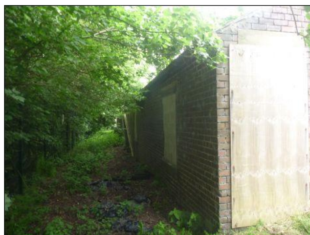
Photo 16: Building 1, south-western elevation
