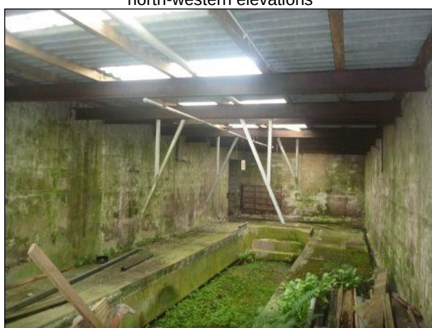
Photo 33: Building 4, section 4.1, internal area
