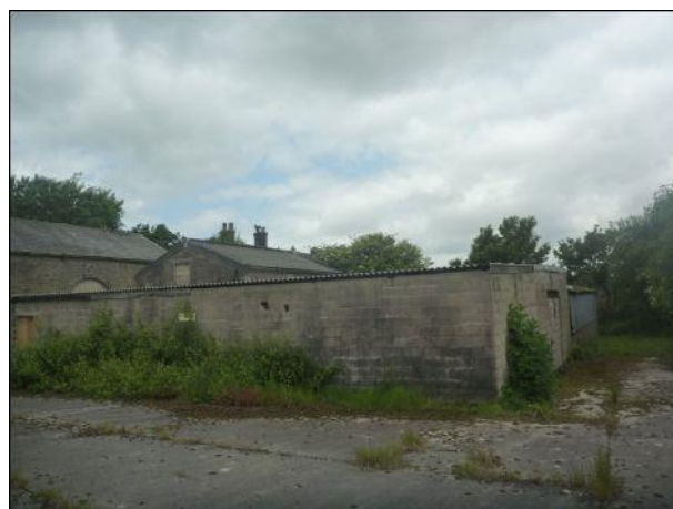
Photo 28: Building 4, section 4.1, south-eastern and north-eastern elevations
