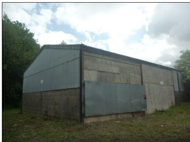
Photo 31: Building 4, section 4.5, south-western and north-western elevations
