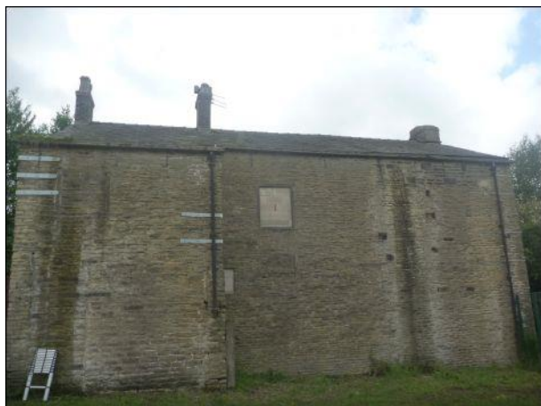
Photo 25: Building 3, north-eastern elevation
