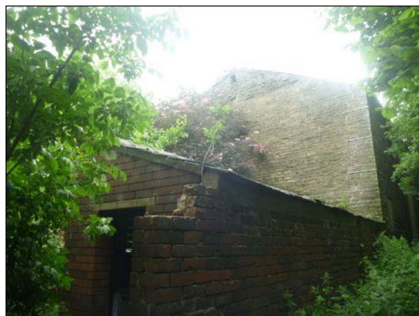
Photo 18: Building 2, north-western gable end and single-storey extension
