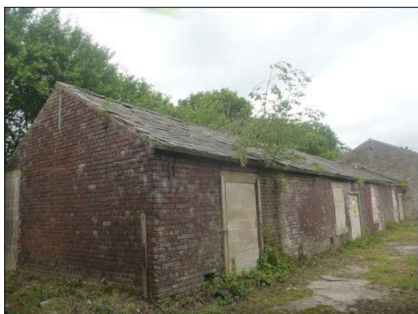
Photo 15: Building 1, south-eastern gable end and north-eastern elevation
