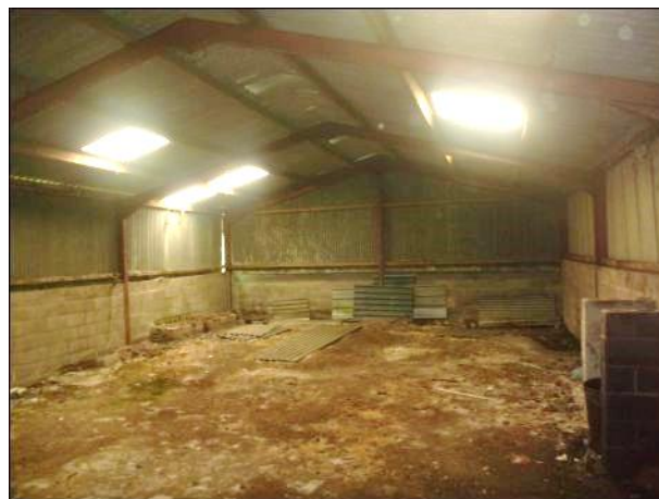
Photo 38: Building 4, section 4.5 internal area
