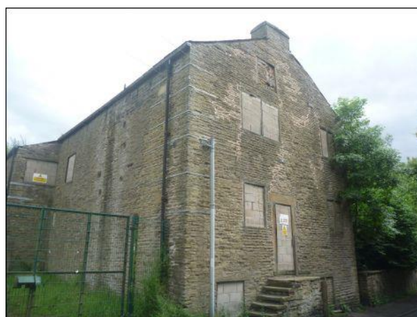
Photo 24: Building 3, north-western elevation
