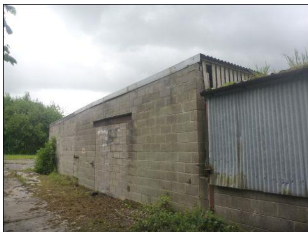
Photo 29: Building 4, section 4.1, north-eastern elevation
