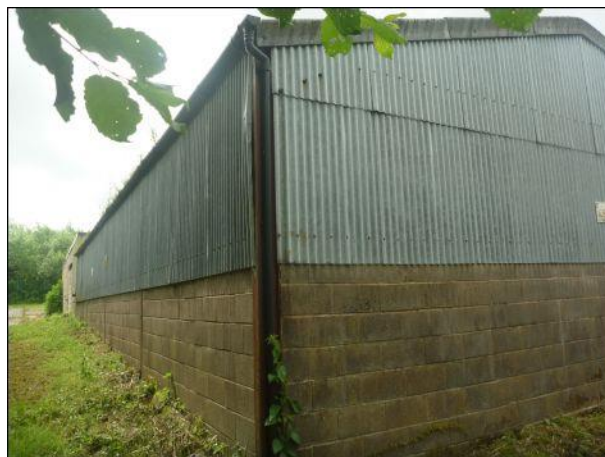
Photo 32: Building 4, section 4.5, north-eastern elevation
