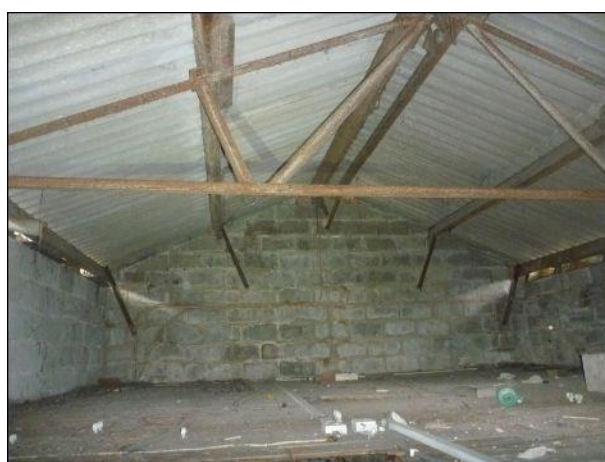
Photo 34: Building 4, section 4.2 roof void
