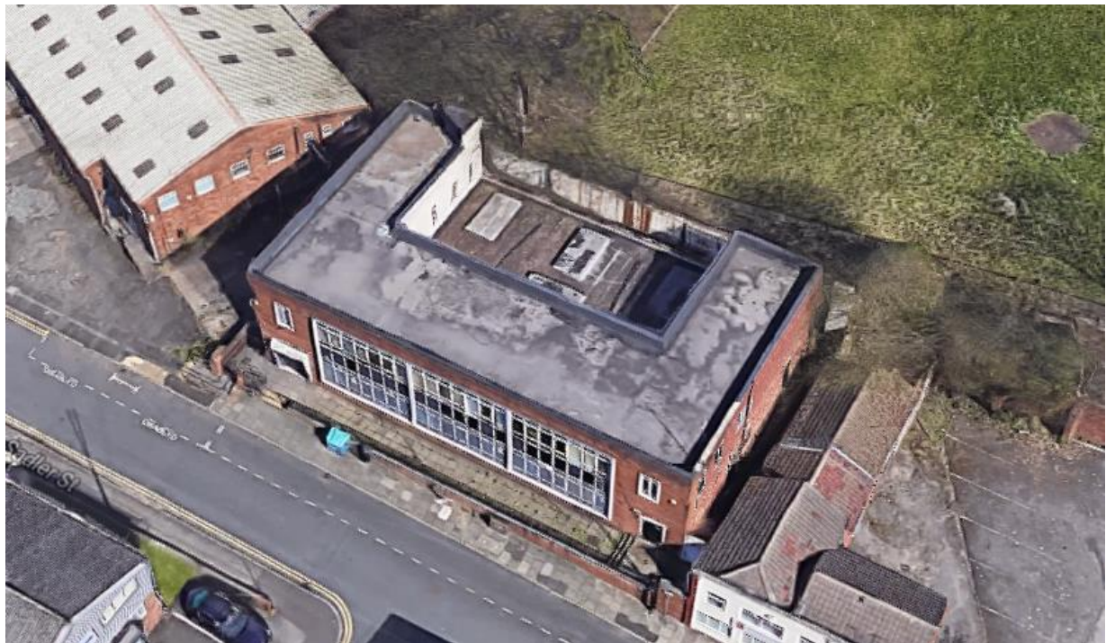
Figure 1: Existing aerial view (Front)
