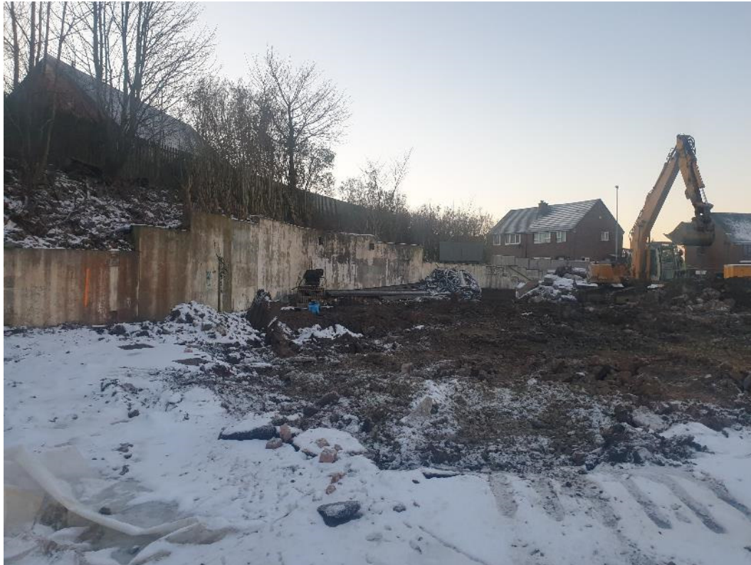
Photograph 3: Footprint of former building following demolition.
