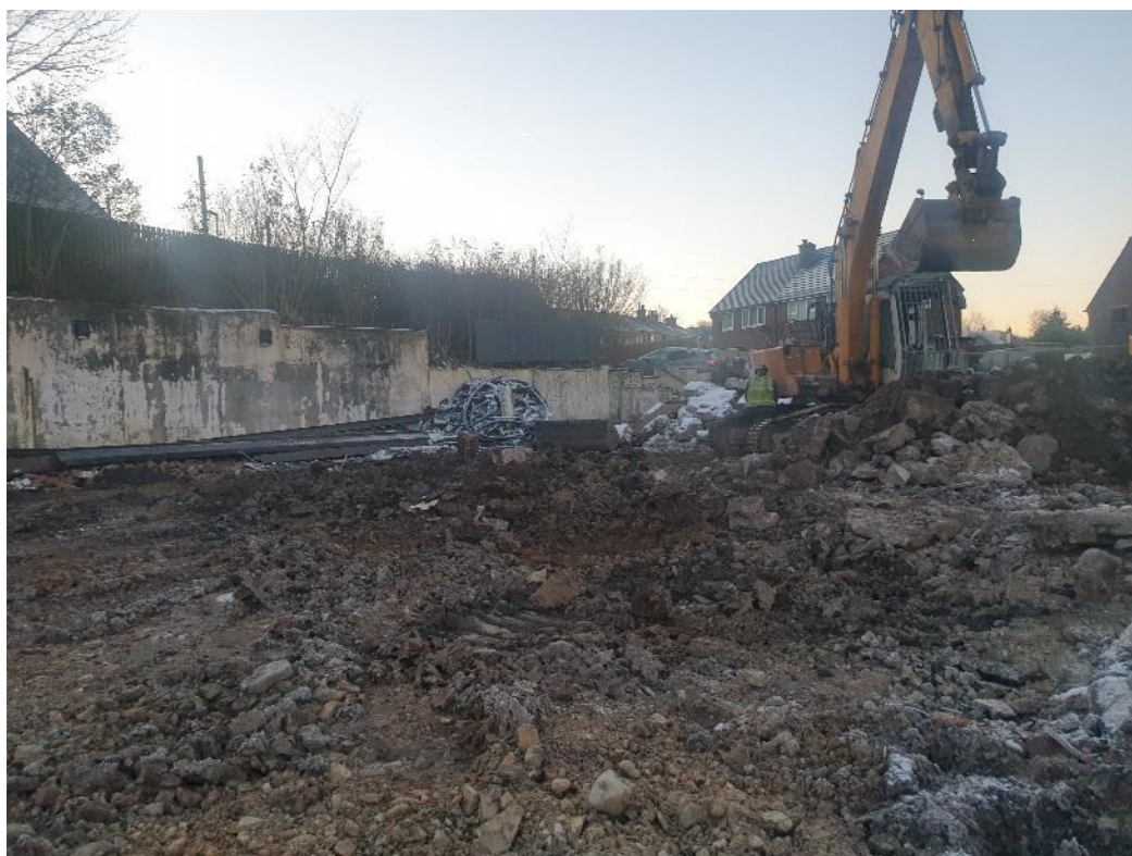
Photograph 1: Footprint of former building following demolition.
