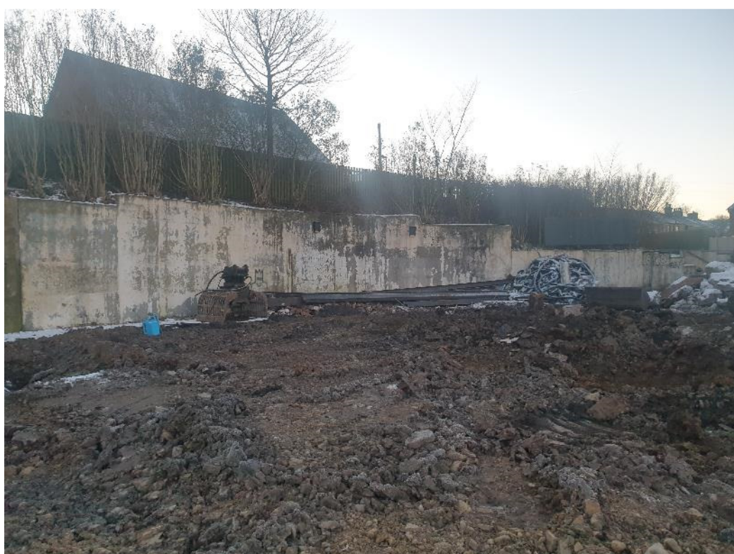
Photograph 2: Footprint of former building following demolition.
