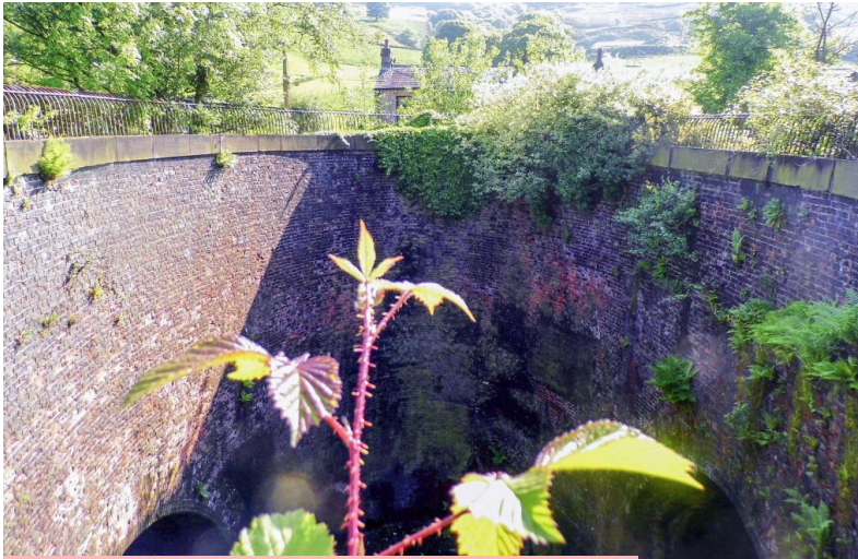
Viewing Oval / Vent – Internal View
