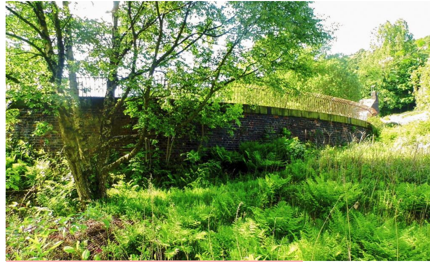
Viewing Oval / Vent – External View
