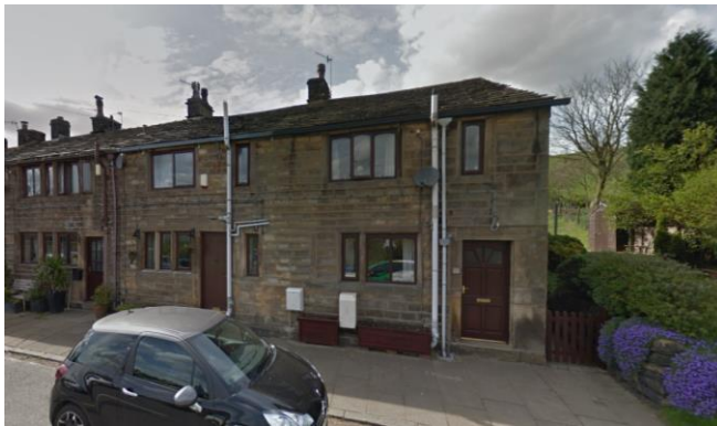
Mews Housing Salley Street
