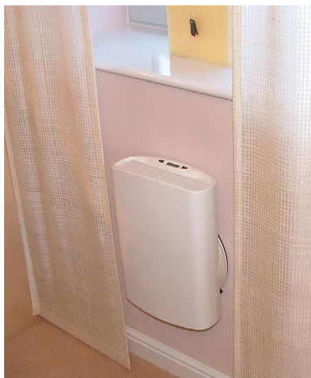
Figure 7 In-situ Titon Sonair acoustic vent
