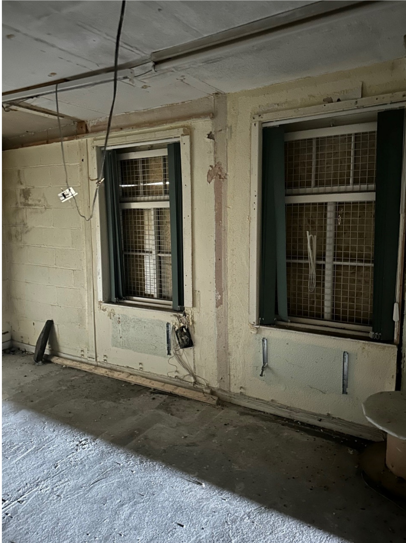
21. Office 4 window detail
