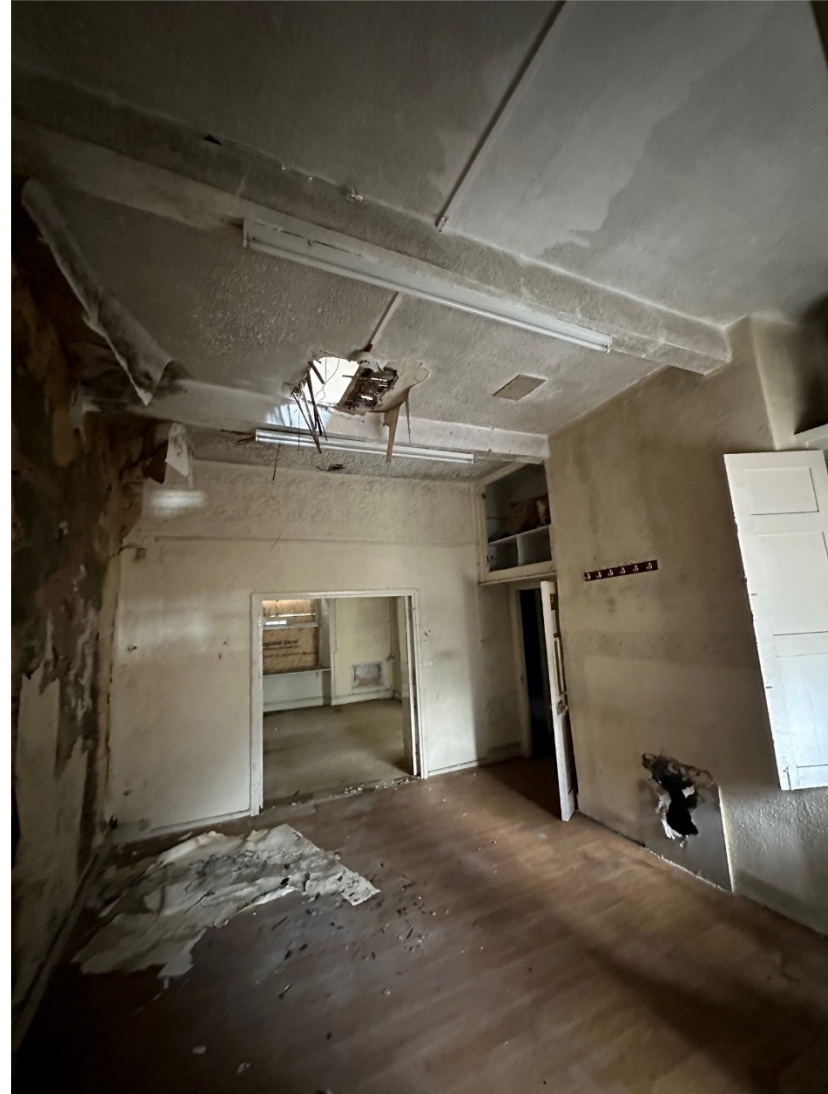
15. Office 2 general view with office 1 in background
