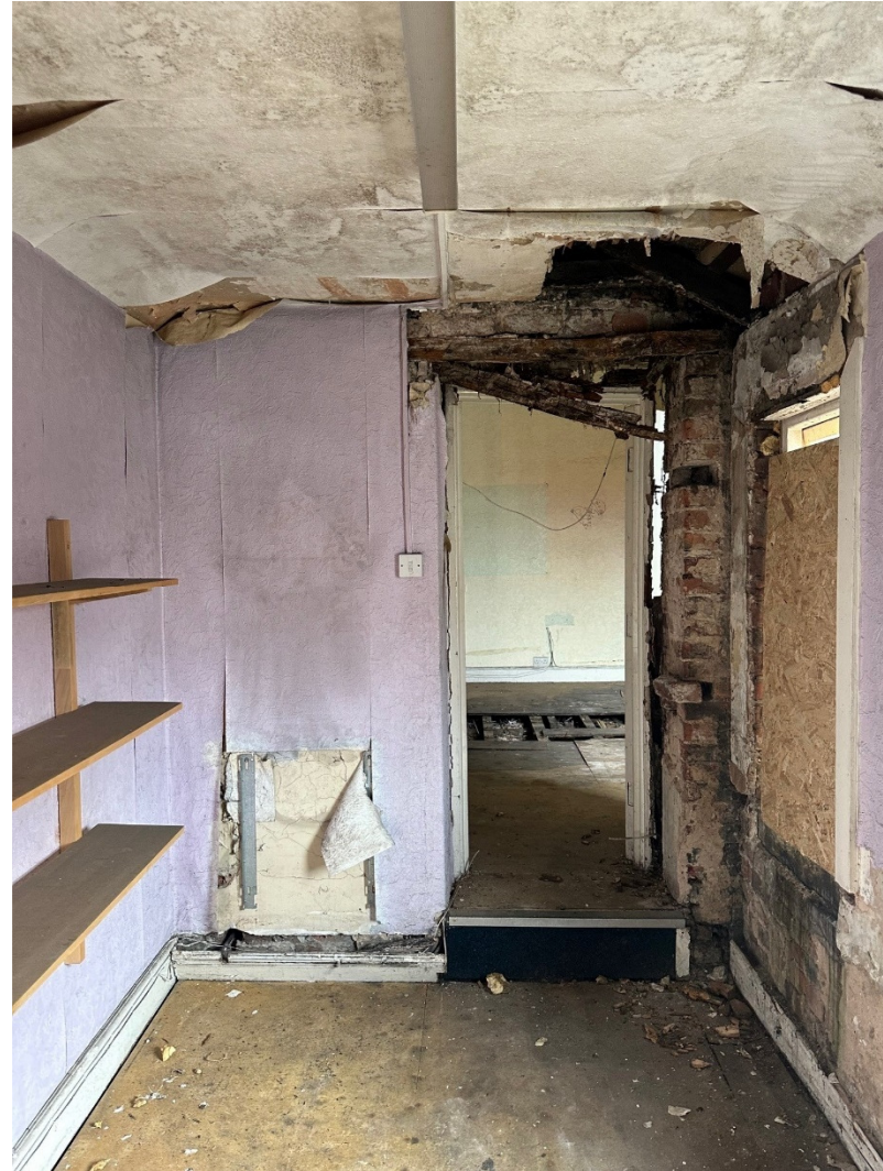
28. Kitchen off office 6
