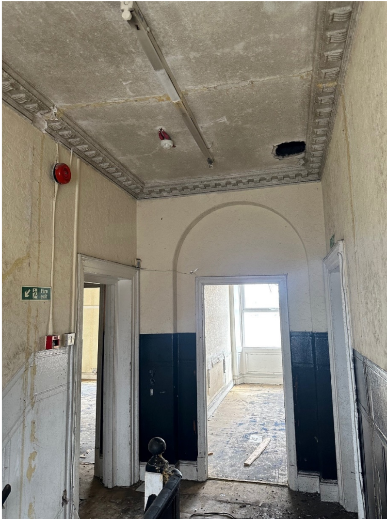
25. First floor landing arch & ceiling detail
