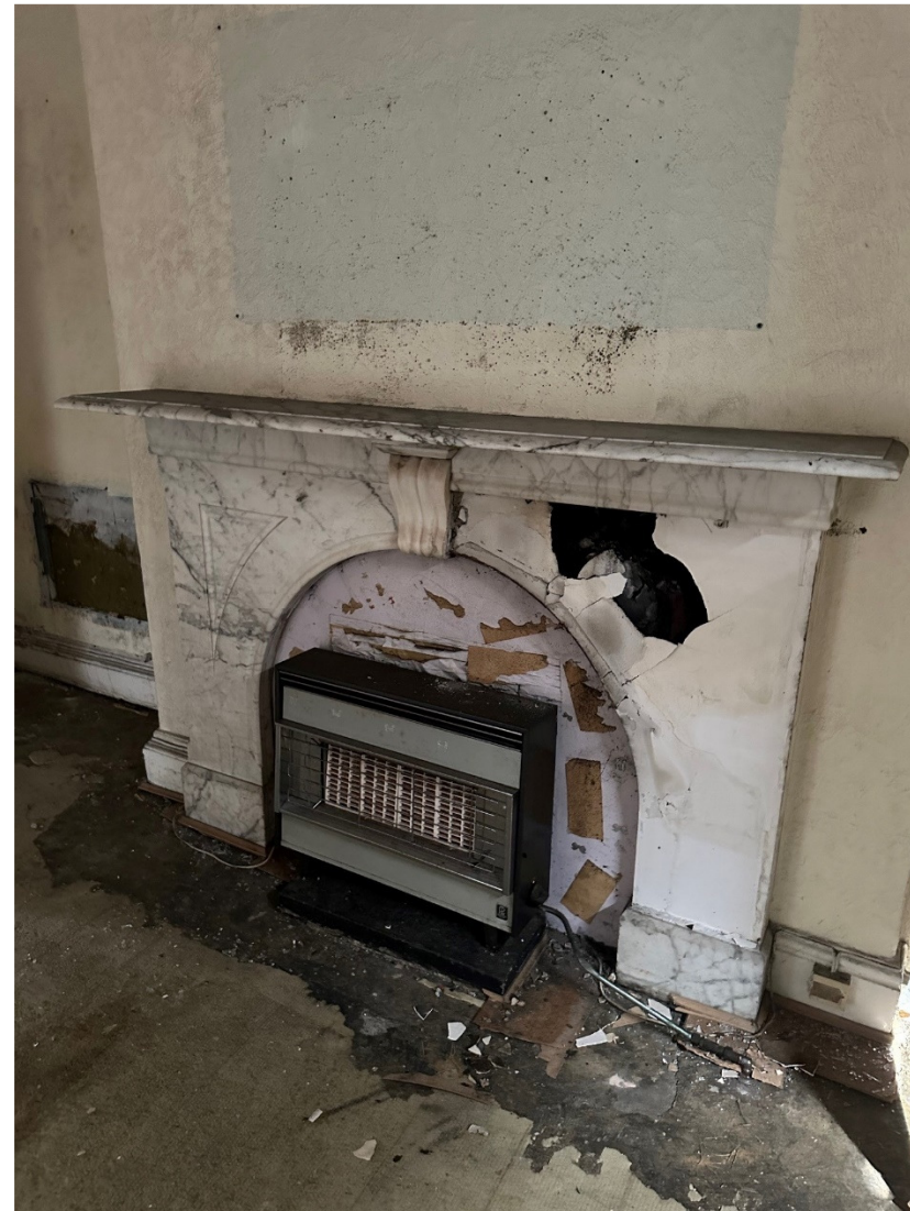
10. Office 1 Fireplace detail
