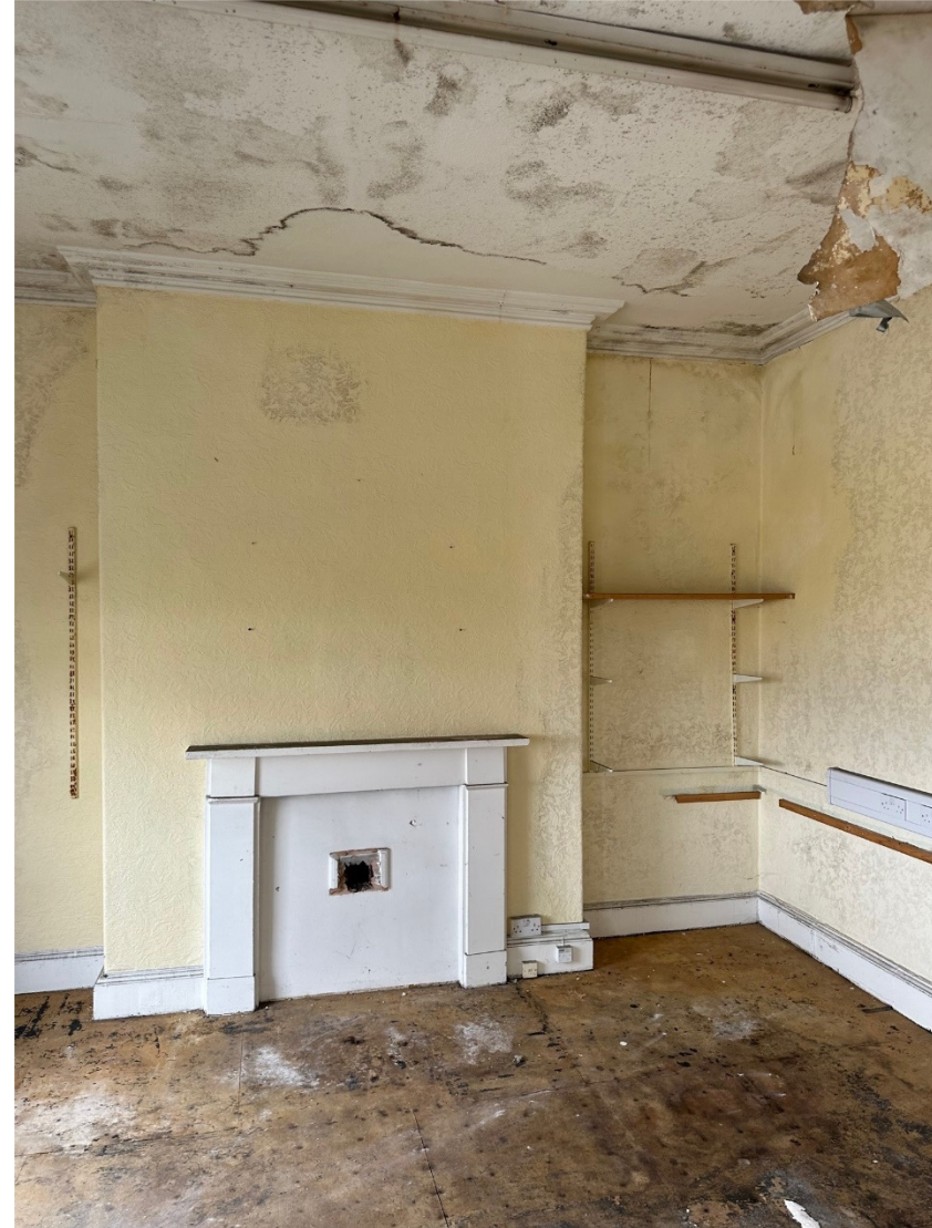
34. Office 8 chimney & ceiling detail
