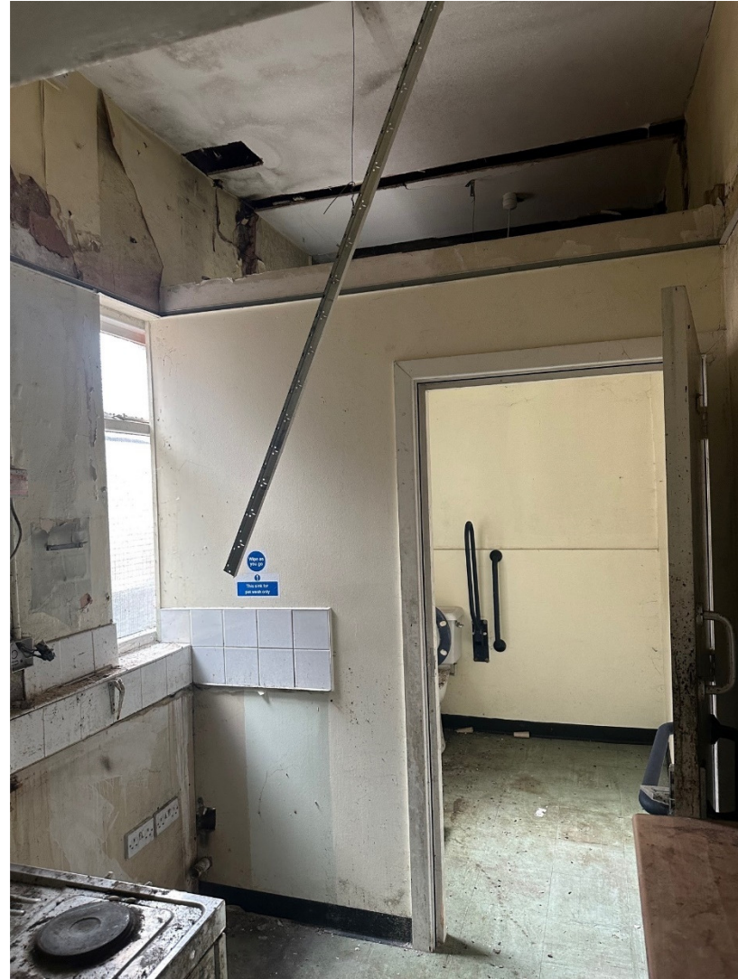
19. Kitchen & WC off office 2
