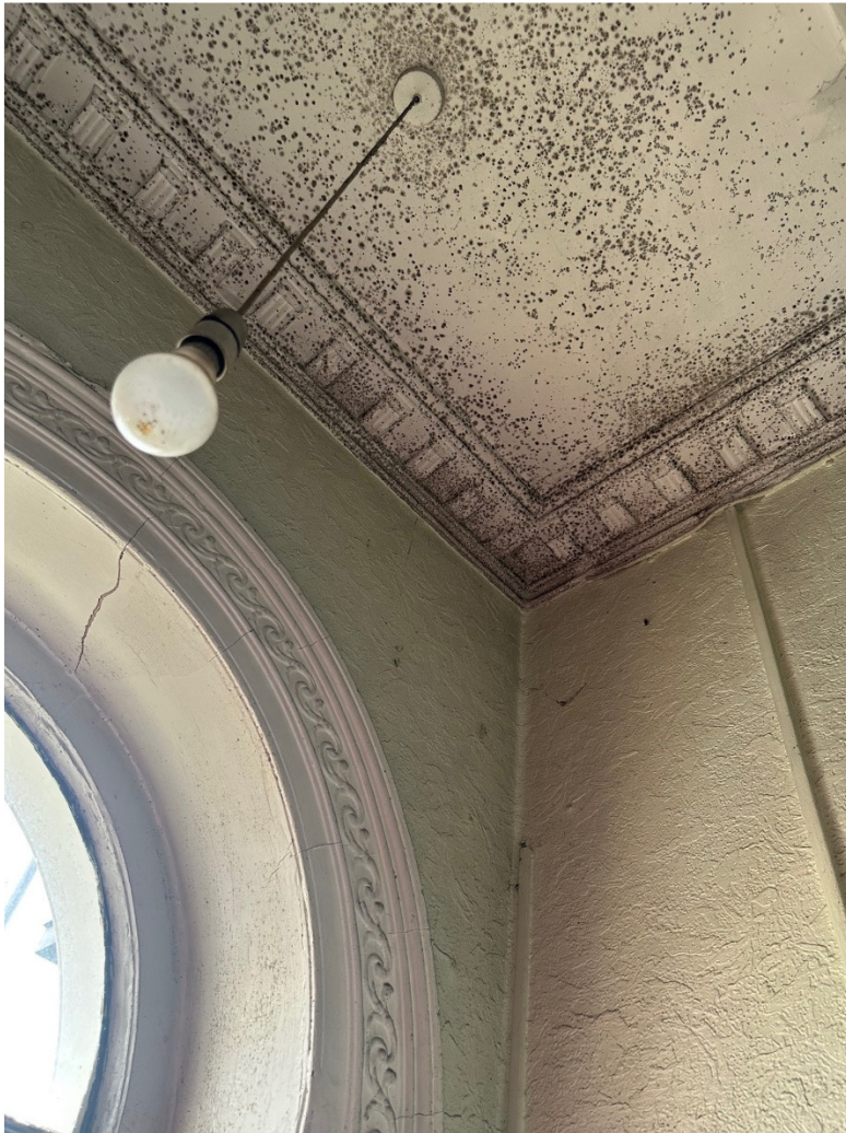
1. Entrance door arch & ceiling
