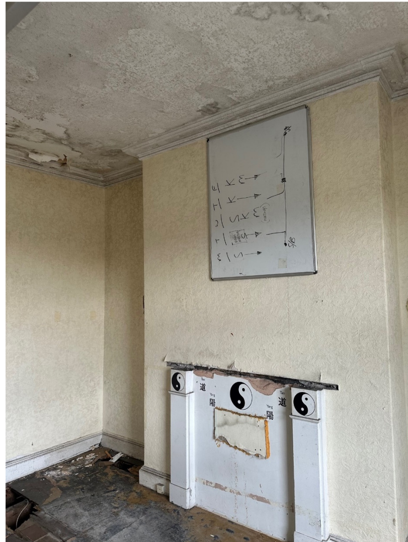
30. Office 7 chimney and ceiling detail
