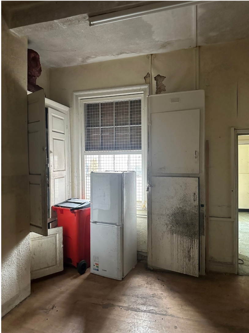
18. Office 2 window & cupboard detail
