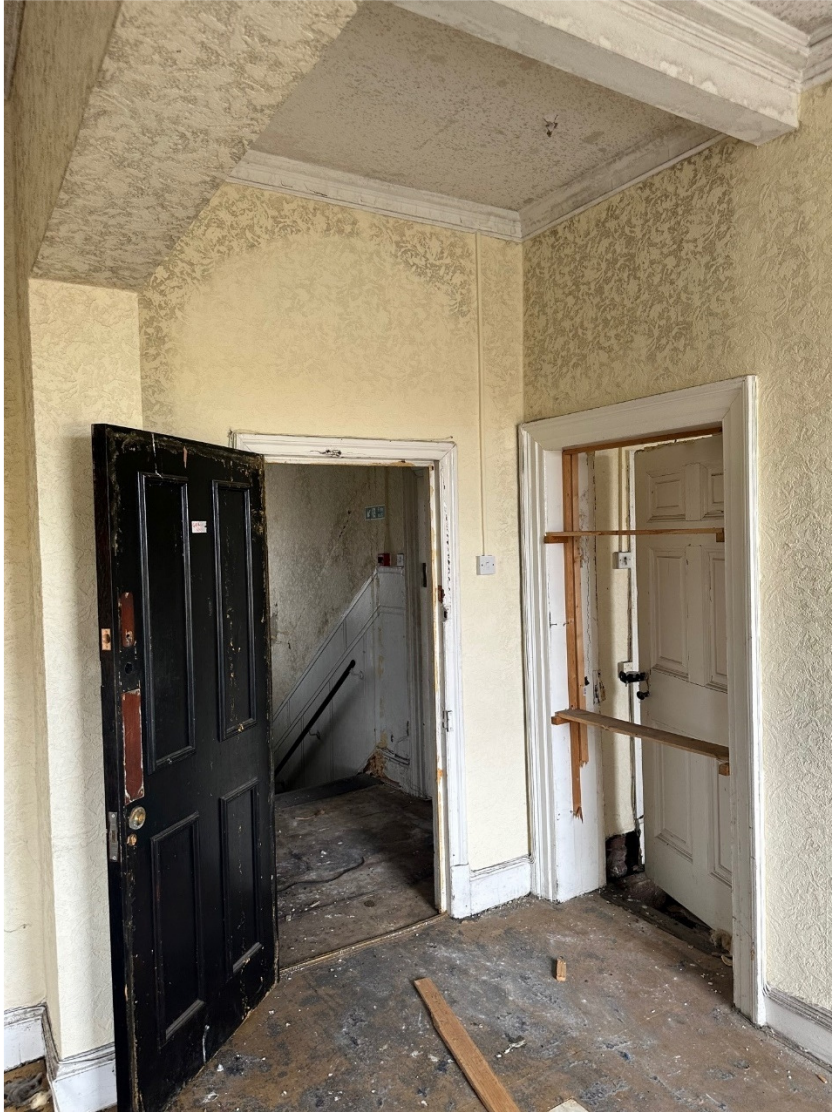
33. Office 8 with door to office 7
