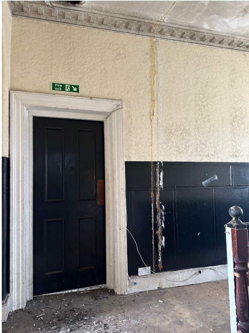
35. Door to office 9 & beyond
