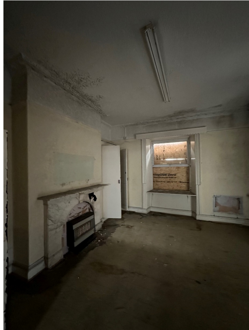
8. Office 1 general view
