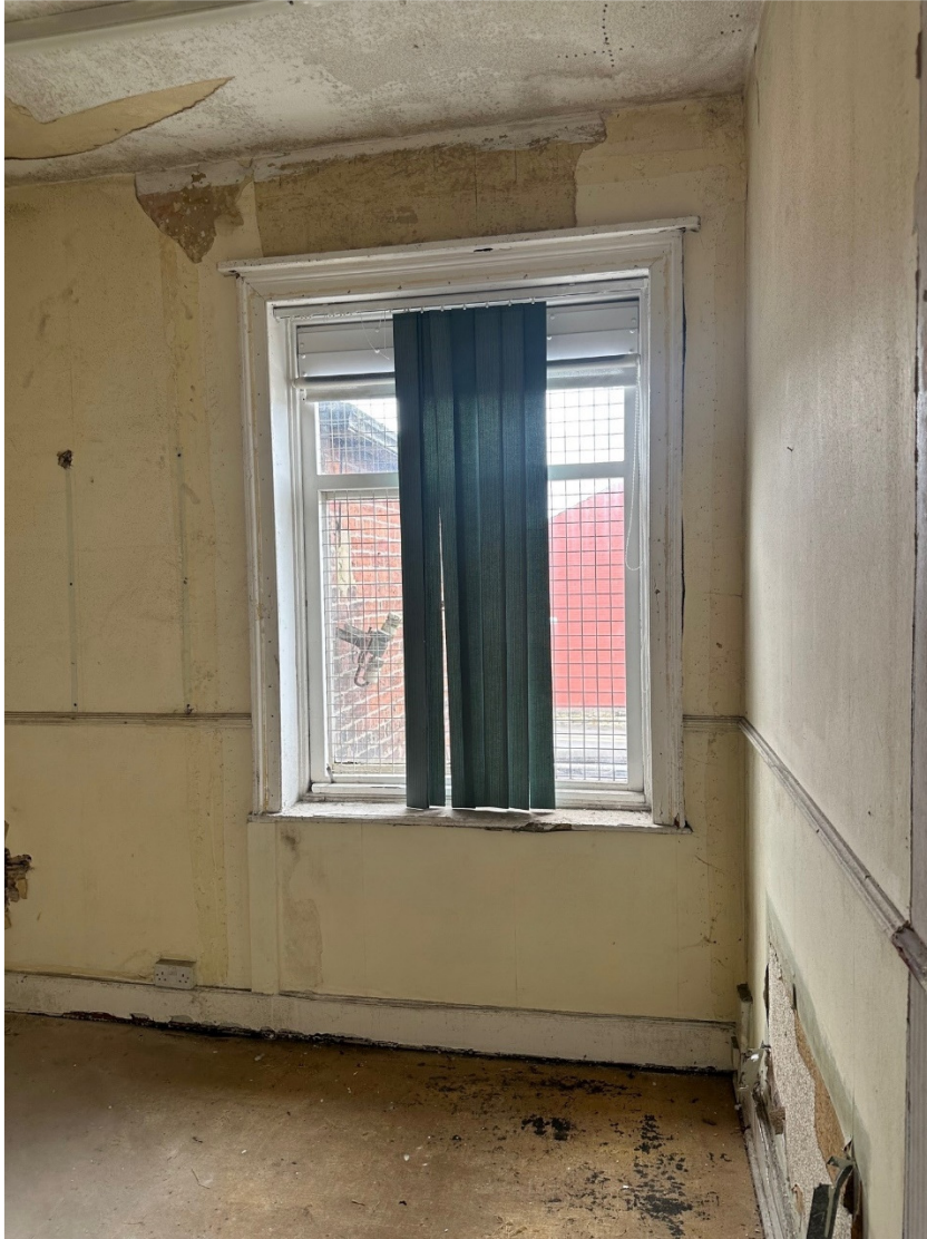
37.Office 9 window overlooking rear yard
