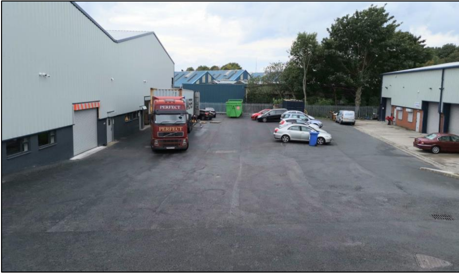
Refurbished commercial units to the south west site.
