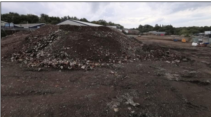
North of the site looking south.
