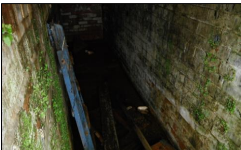
Service trench (Building 3 to N of Site).
