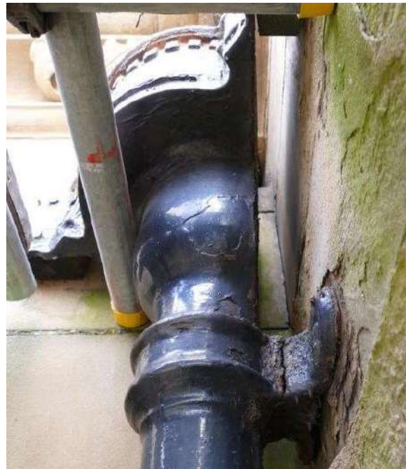
Fractured ear band, corroding fixings and spalling finishes. Repeated saturation of the adjacent masonry has led to extensive spalling and algae growth. The gully was blocked when surveyed.
