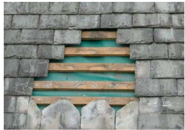
Opened up area reveals breathable felt, battens, fixings and slate all to be in good condition.
