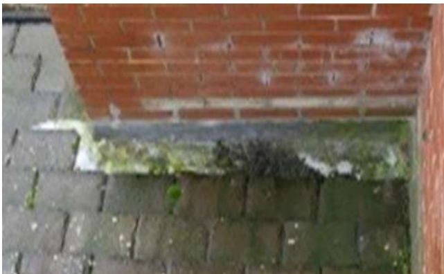
Narrow back gutter flashings to adjacent roof and limited outfall. Lack of fall and debris leading to standing water and potential rot of timbers below.
