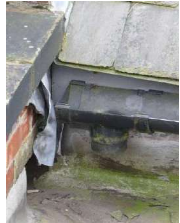
Opened weathered joints in the copings
