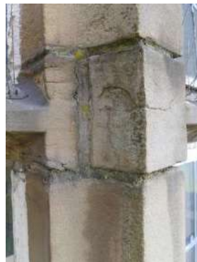
Spalling facings and past cementitious pointing..
