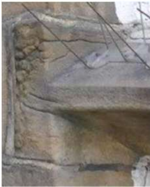
Spalling facings and past cementitious pointing..
