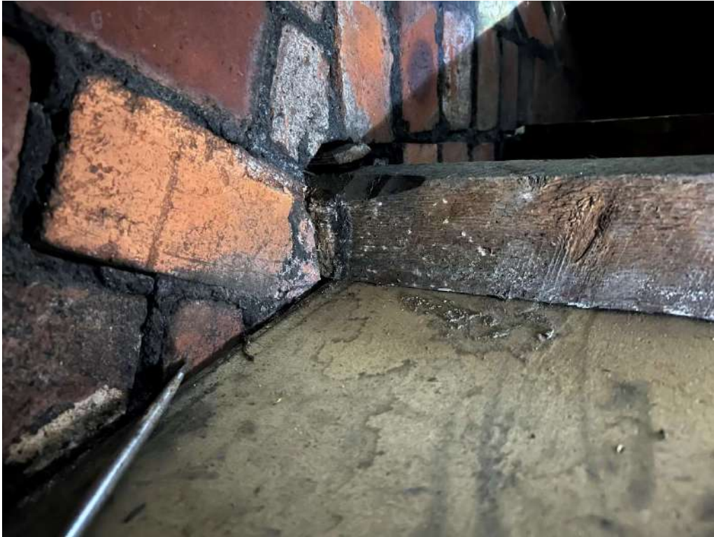
Ceiling joists and purlin above curved ground floor library ceiling Photo 2
