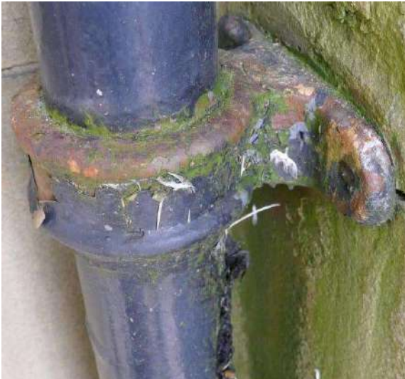
Fractured ear band, corroding fixings and spalling finishes. Repeated saturation of the adjacent masonry has led to extensive spalling and algae growth. The gully was blocked when surveyed.
