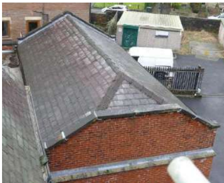
Library roof with concrete ridge tiles and welsh blue and heather slates
