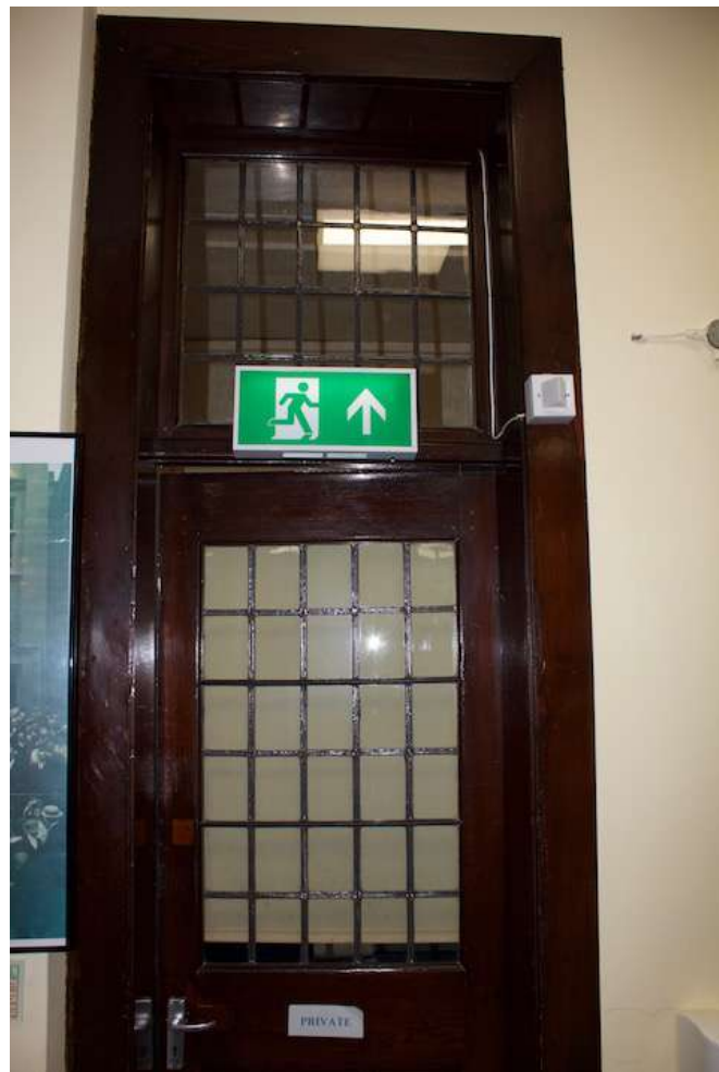
Door to staff room
