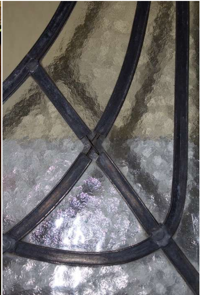
Example of broken solder
