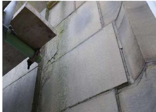
Line of displacement of masonry by the oriel window..
