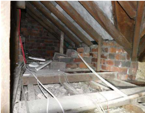
Void below the oriel roof area
