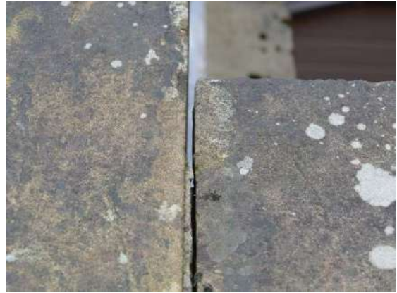
Opened weathered joints in the copings
