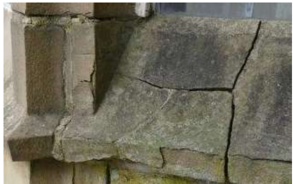
Line of displacement of masonry by the oriel window..
