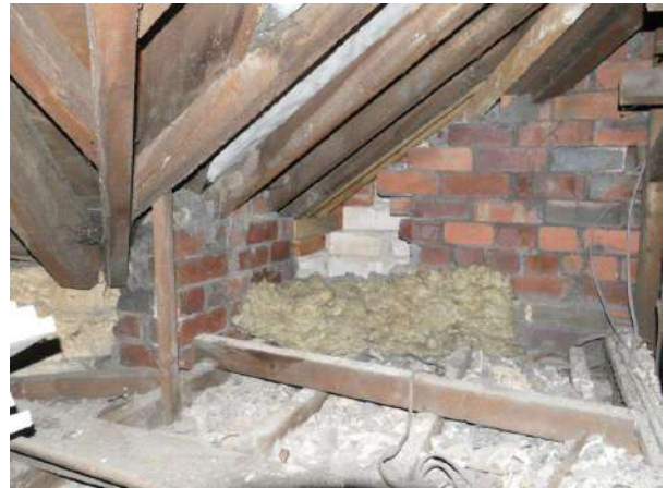
Roof void above Oriel window projection
