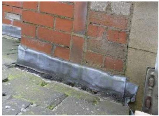
Narrow back gutter flashings to adjacent roof and limited outfall. Lack of fall and debris leading to standing water and potential rot of timbers below.
