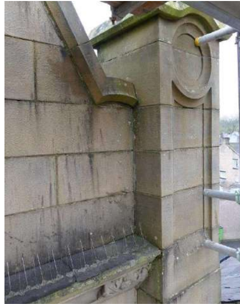
The south pier and finial has a distinct lean to the south which has further opened the joint to the gable panel
