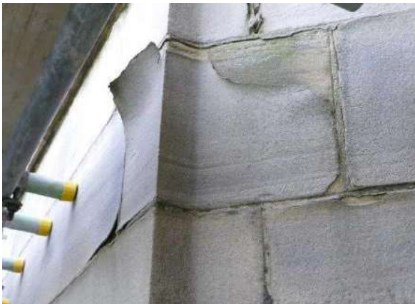
Spalling facings and past cementitious pointing..
