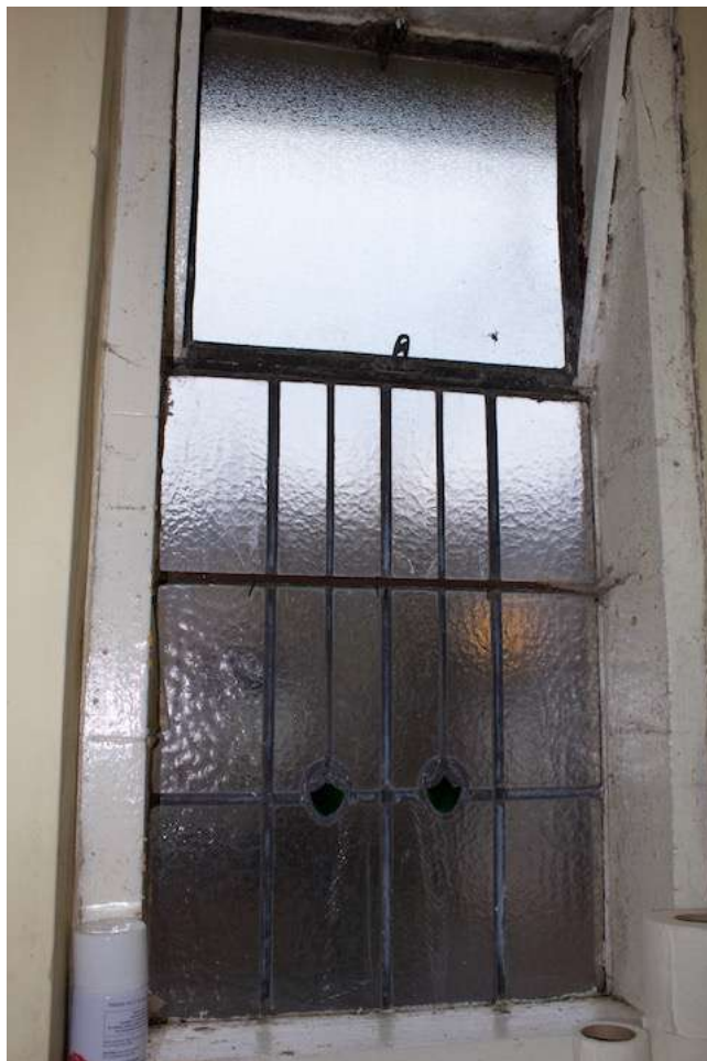
Toilet window internal
