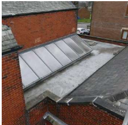
Opened weathered joints in the copings
