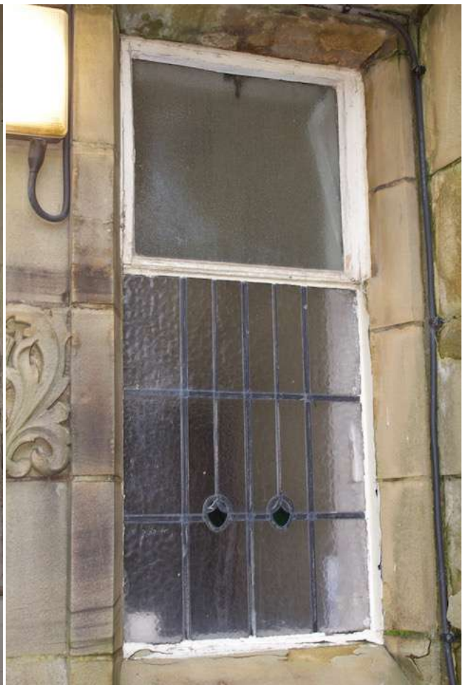
Toilet window external
