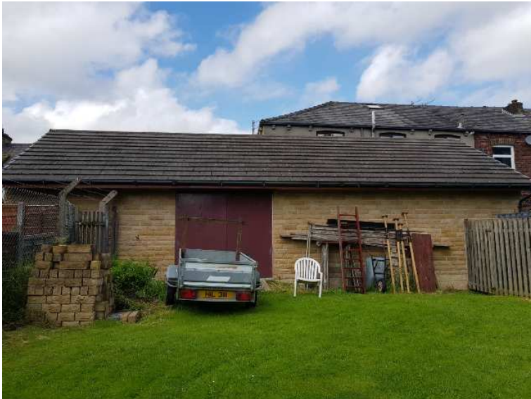
Rear view of garage
