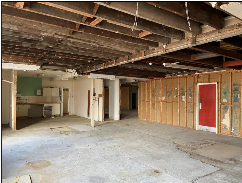
Photograph 5 showing the interior of the first floor
