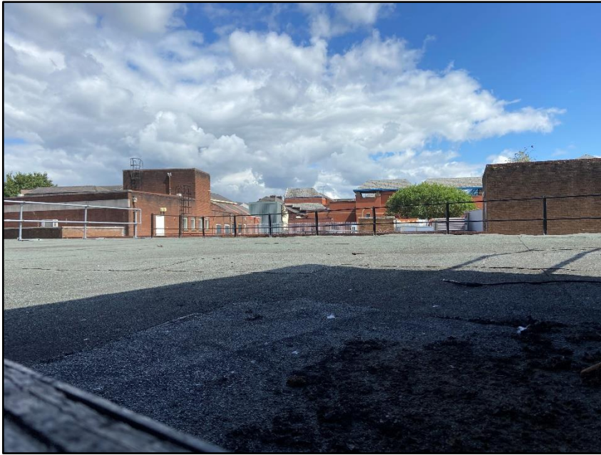
Photograph 4 showing the flat roof
