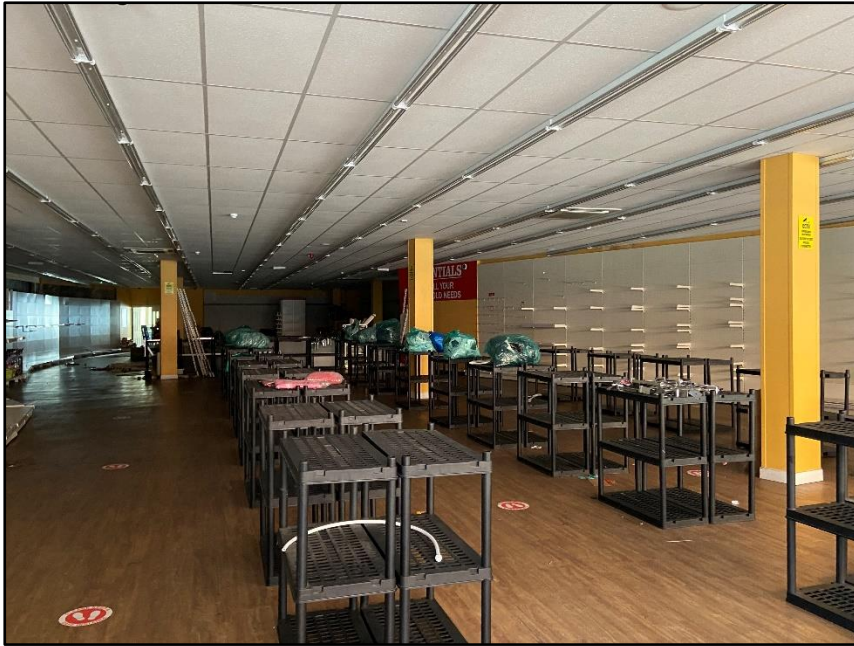
Photograph 6 showing the interior of the ground floor
