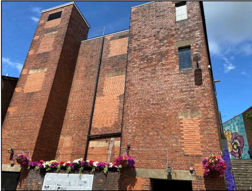
Photograph 2 showing the rear of 46 Yorkshire Street
