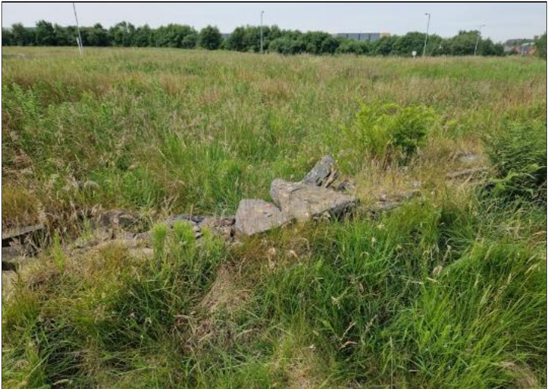
Photo 10—Western section of site, old drystone wall that runs across the site from west to east.
