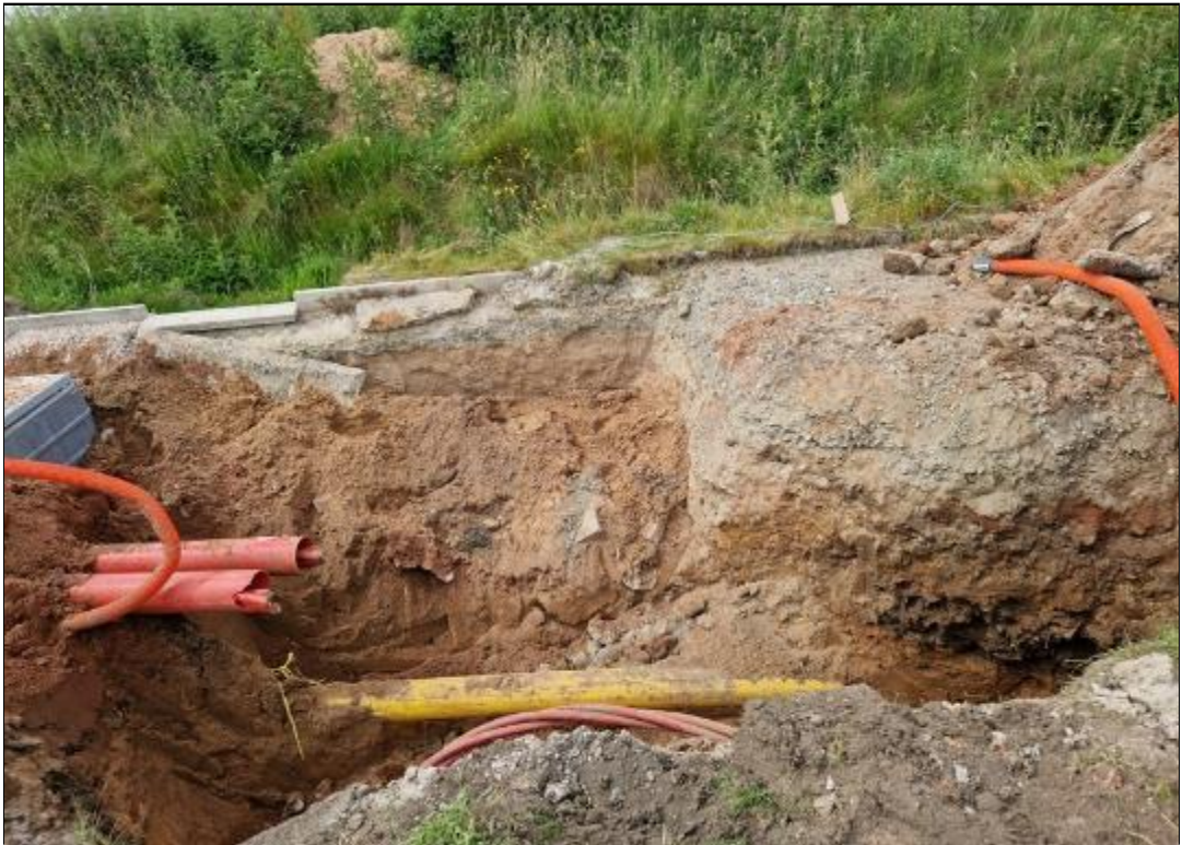
Photo 3—Opposite footpath towards the south, open utilities excavation across the road
