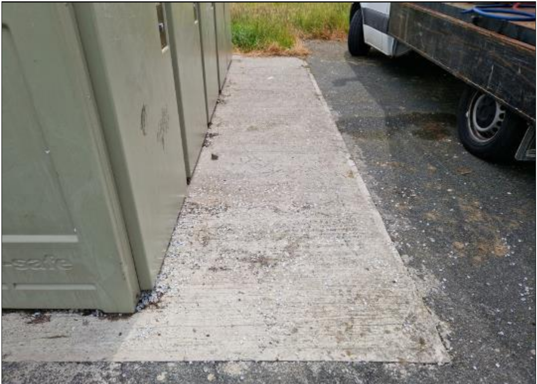
Photo 9—Broken glass alongside bicycle storage
