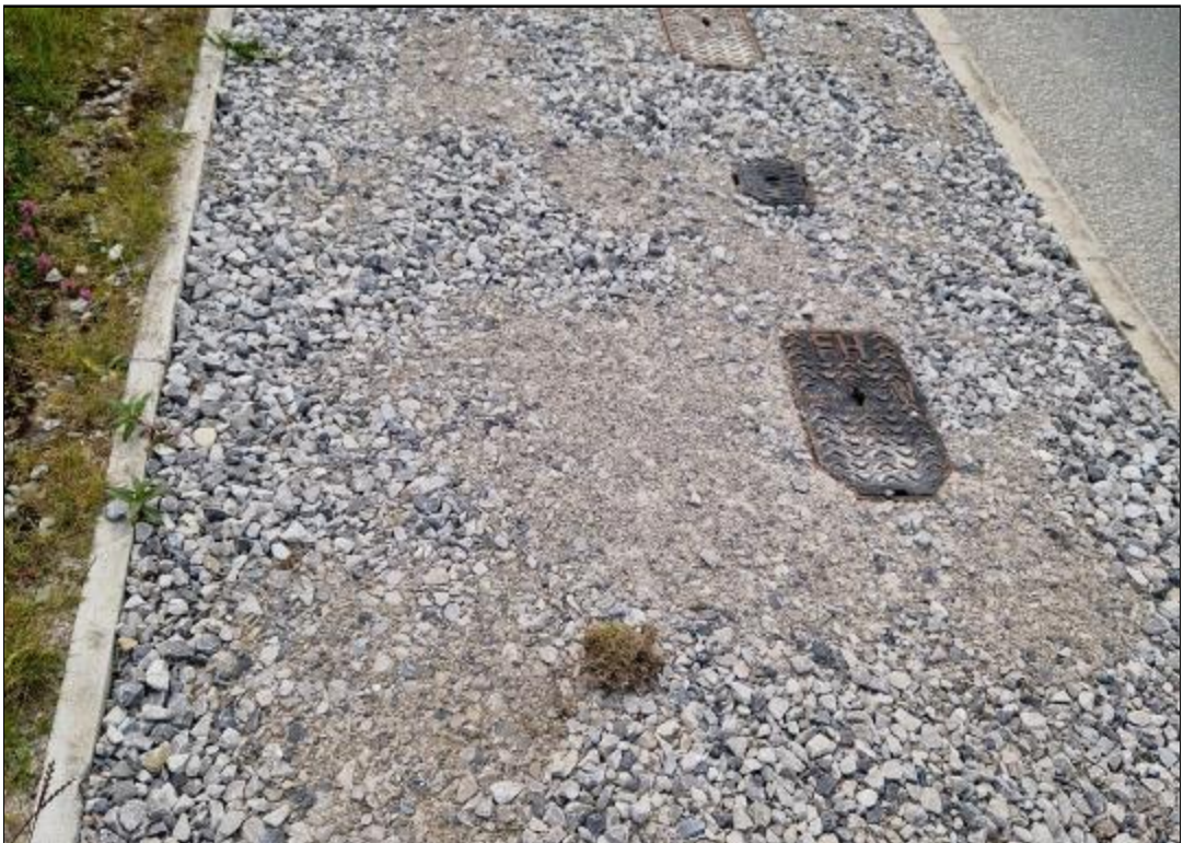
Photo 16— On northern pavement of tarmac road are utilities accessible for site work
