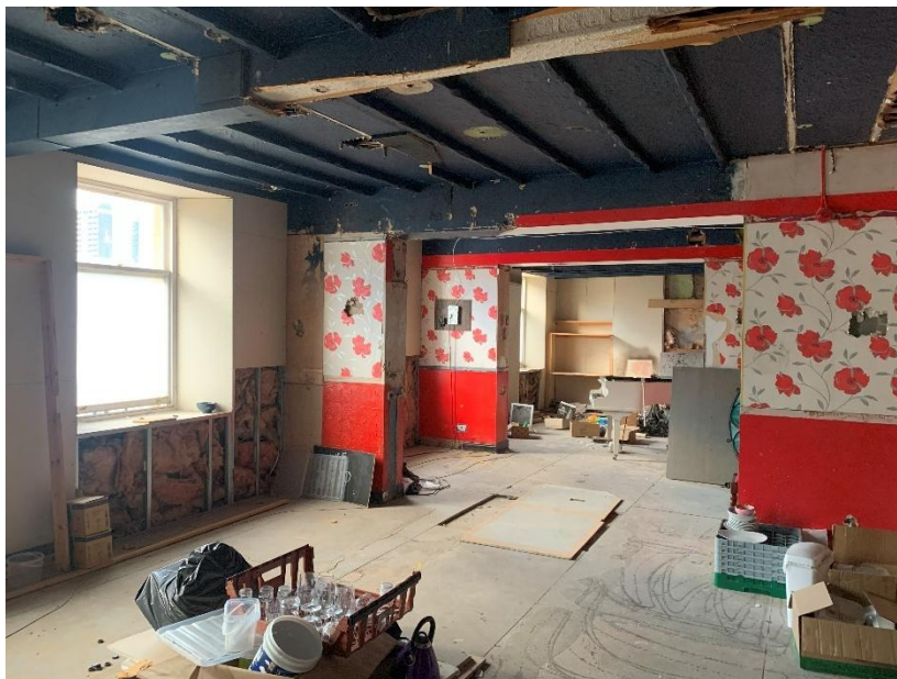
Figure 2.4: view of first floor showing removal of internal walls.
