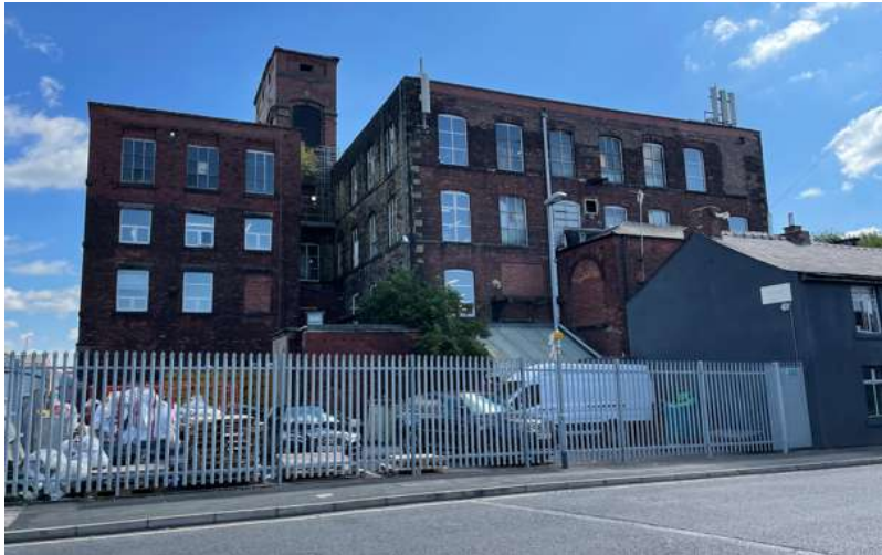
Figure 4.3: View from Whitehall Street / Princess Street (2022)
