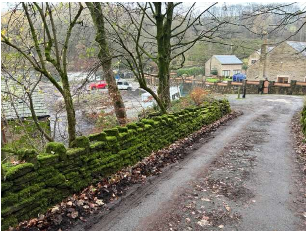
Plate 12 – View towards site from access leading up to Huddersfield Road
