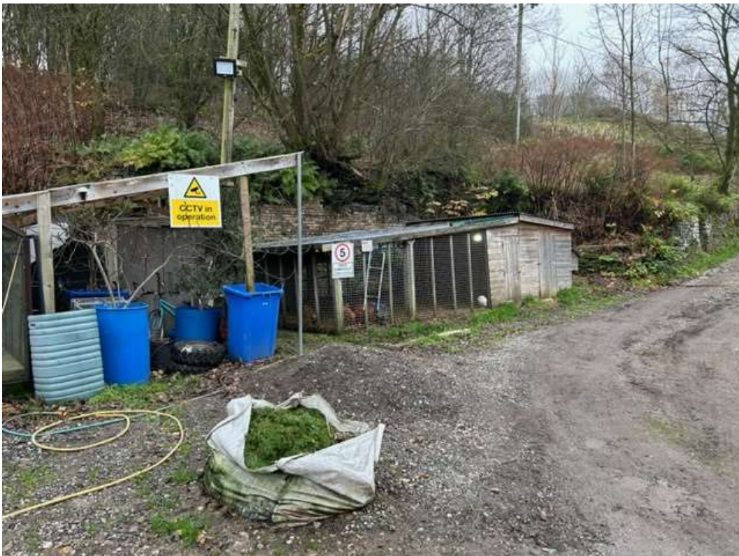
Plate 8 - Retaining wall from Mill development at south east of site
