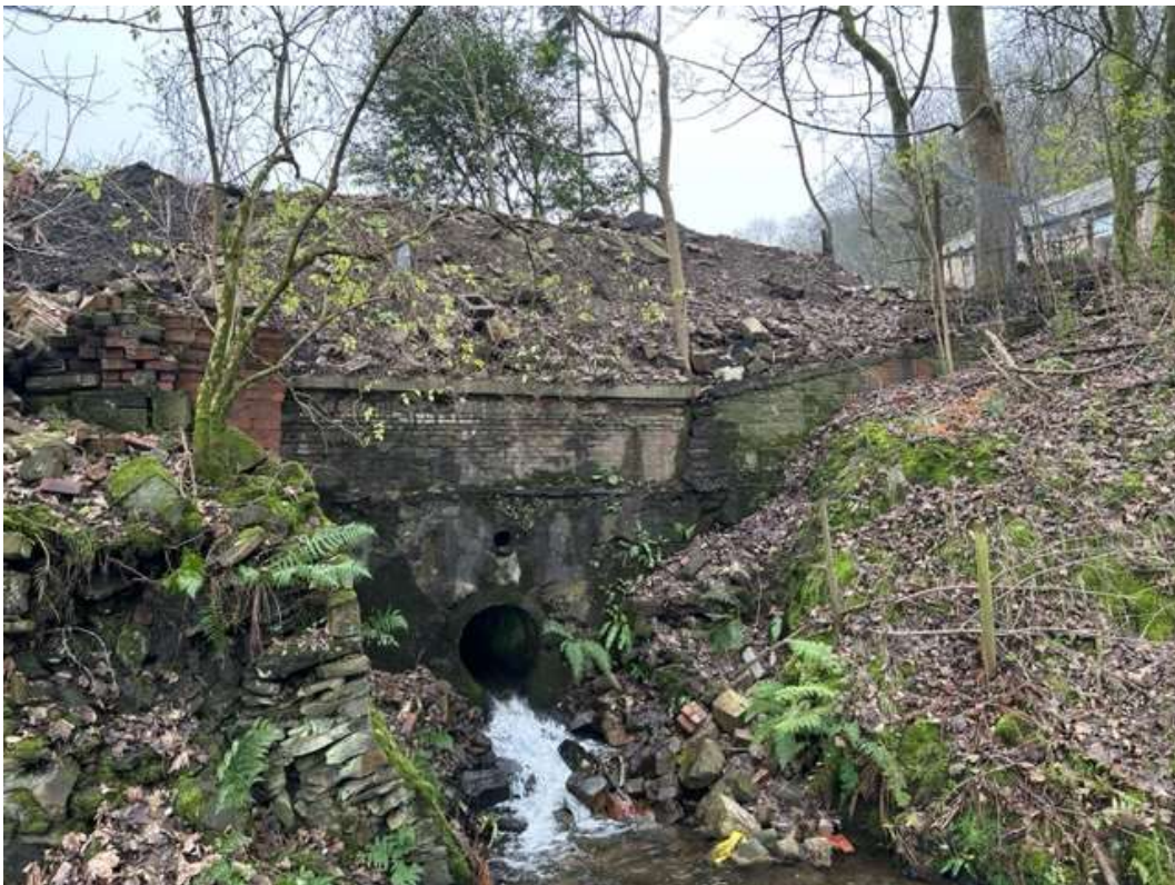
Plate 16 – Mill retaining wall and culvert discharge at north boundary
