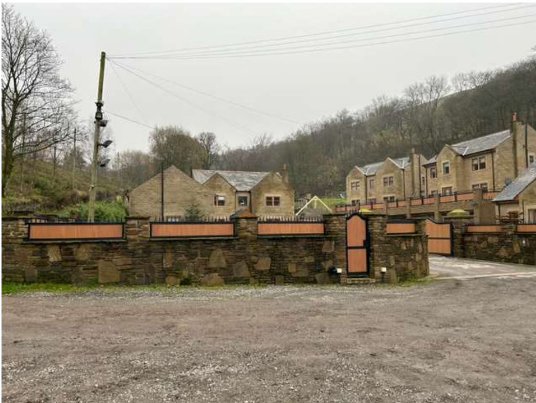
Plate 4 – View from subject site to Carp View development
