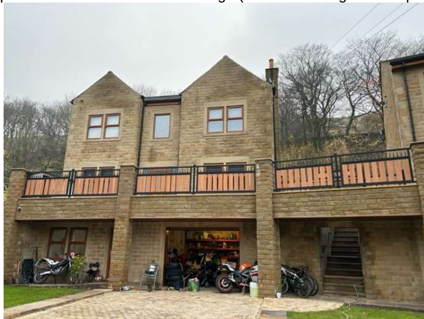
Image 5 – Three storey build at Carp View
