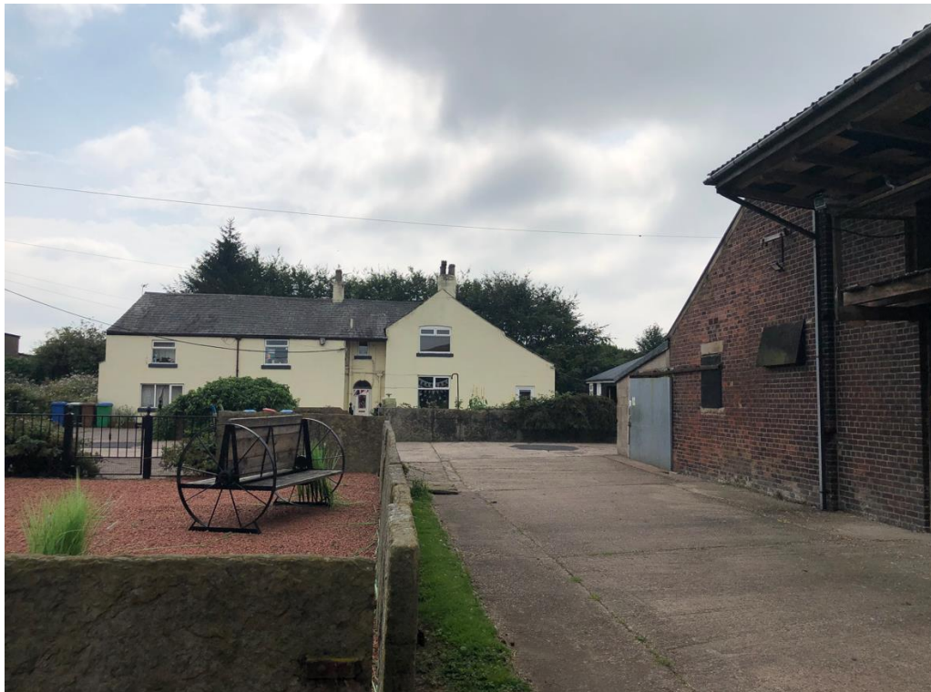
Figure 4.4: Principal (north) elevation of Lower Whittle Farmhouse with 19 th century stables (right of image)
