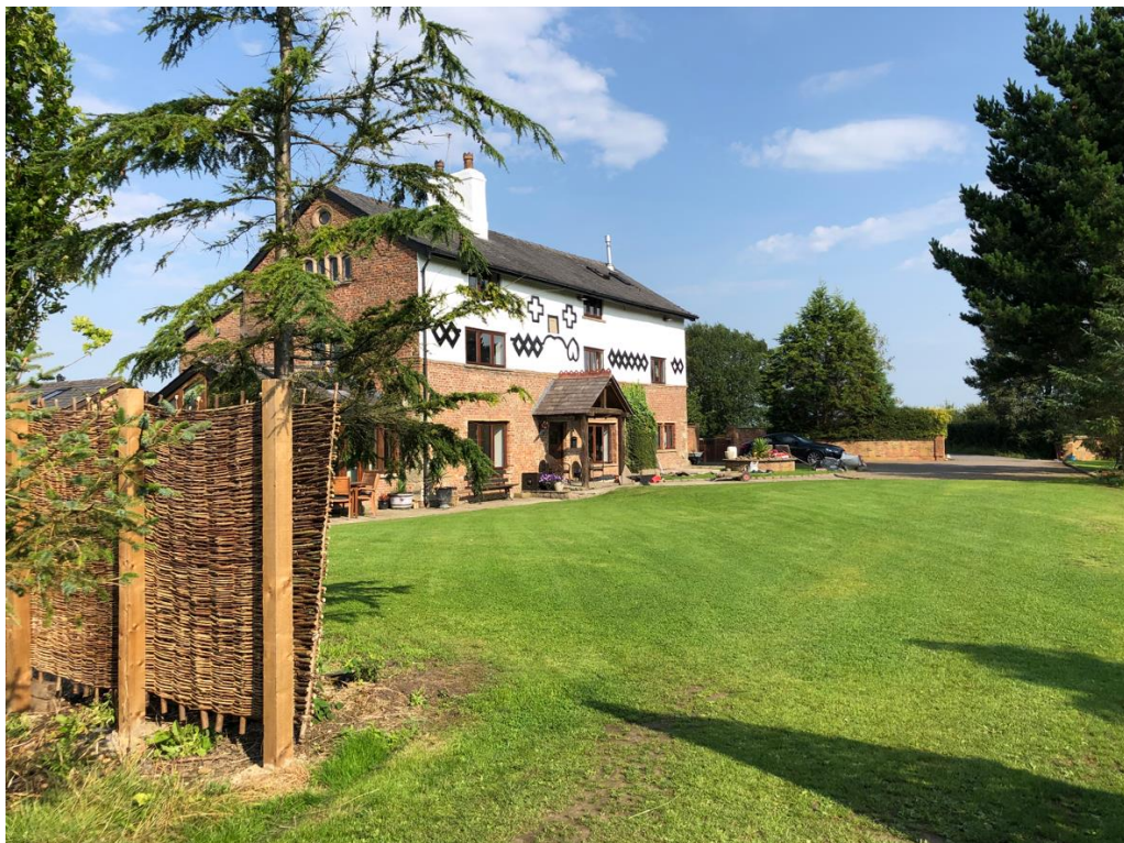
Figure 4.1: Brick House Farm, view of its principal (east) elevation, looking north
