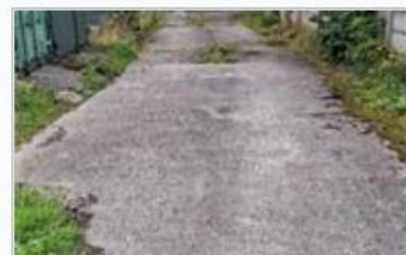
No visible signs of JKW growth in this area at the time of visit
