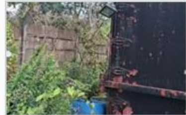
JKW02 between building and fence line
