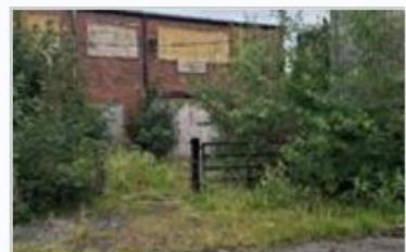
No visible signs of JKW growth in this area at the time of visit
