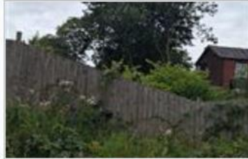
JKW growth noted off site
