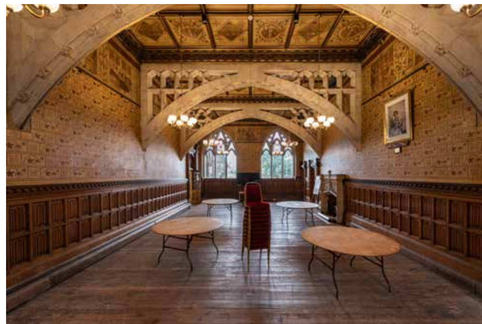
2.6 Traceried stone beams in the former Council Chamber, G1b (Damian Griffiths 2019)
