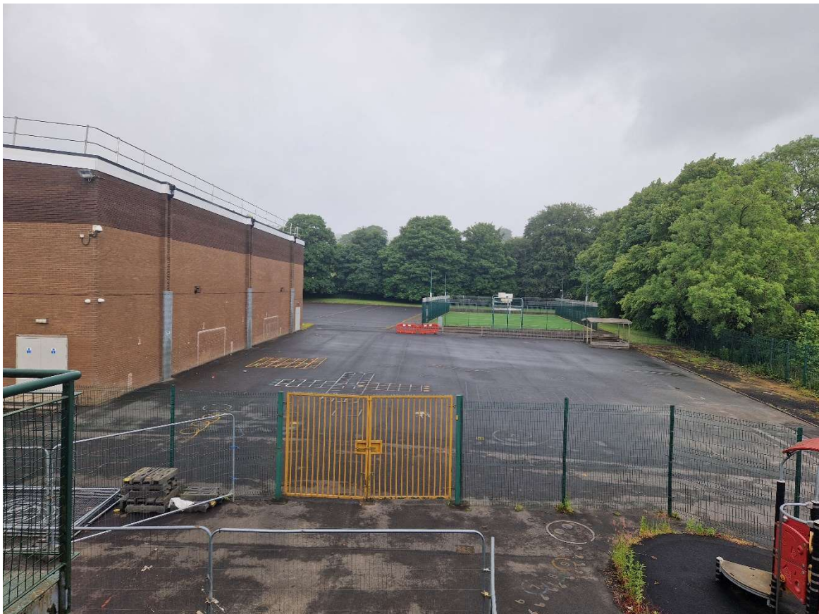
Photo taken from the metal 1 st floor fire escape staircase on the existing building, North Elevation. Town House is adjacent to the MUGA in the distance, which is screened by the trees, hedges and a 2.4m high fence on the boundary.
