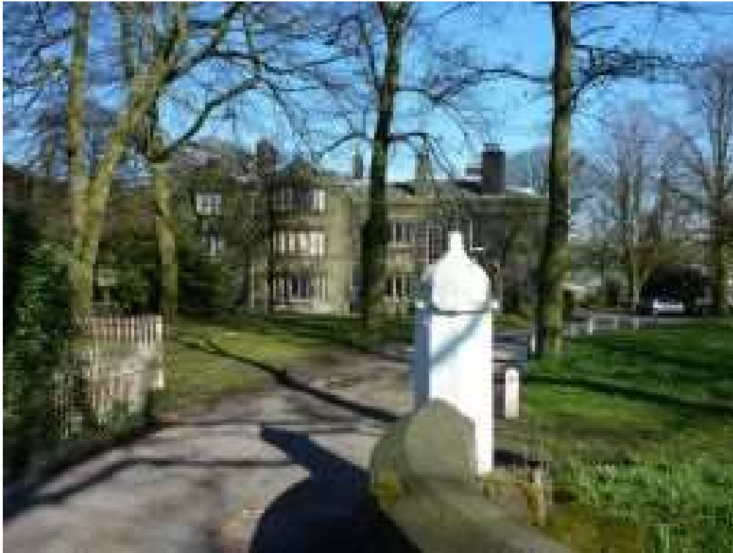
Town House – Grade 2 Listed building in the Conservation Area. Set back and screened by trees and is 126m from the proposed work on the existing building.
