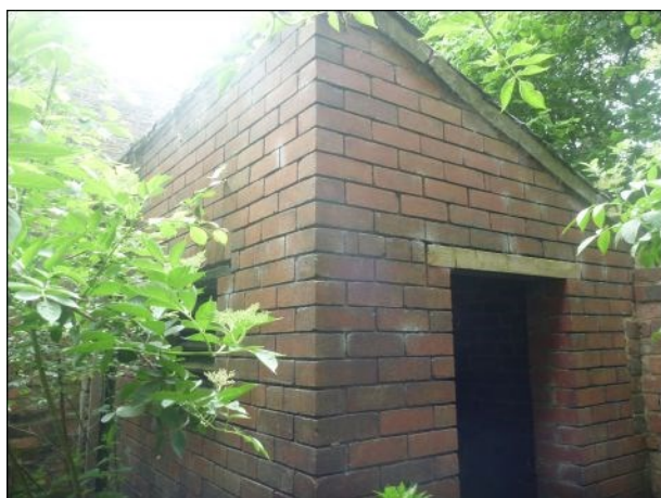
Photo 19: Building 2, single-storey extension
