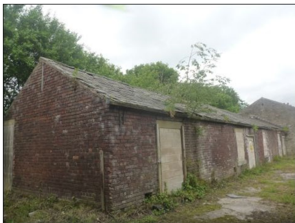
Photo 15: Building 1, south-eastern gable end and north-eastern elevation
