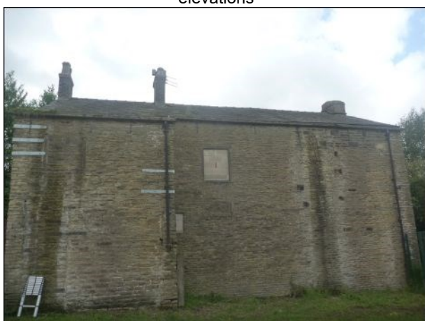
Photo 25: Building 3, north-eastern elevation
