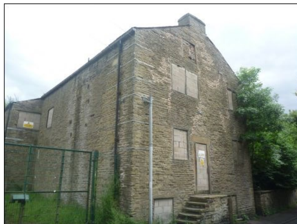
Photo 24: Building 3, north-western elevation
