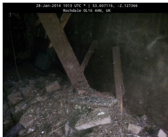
Photo 20: Building 2 internal area (photograph taken in 2014 and provided by the client)
