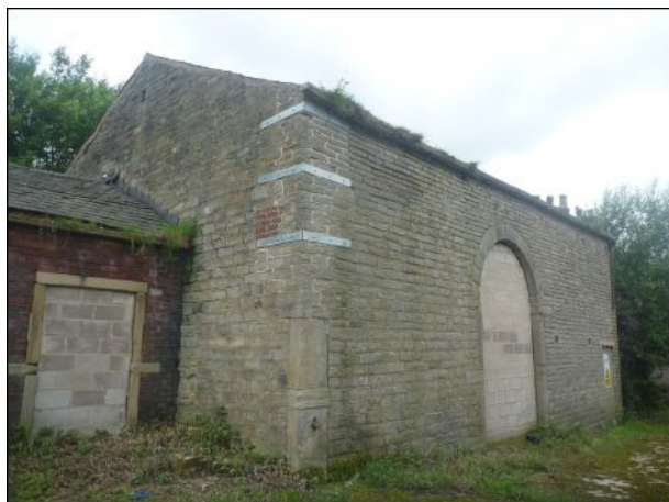
Photo 17: Building 2, south-eastern gable end and north-eastern elevation
