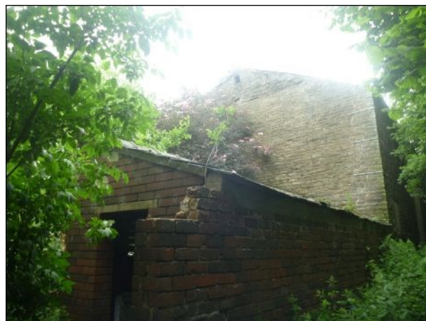
Photo 18: Building 2, north-western gable end and single-storey extension
