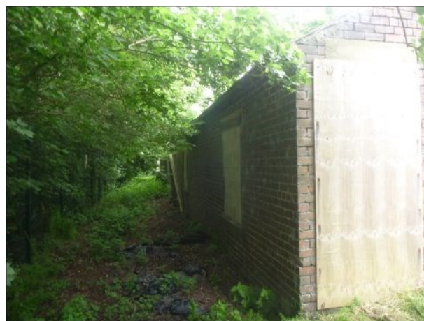
Photo 16: Building 1, south-western elevation
