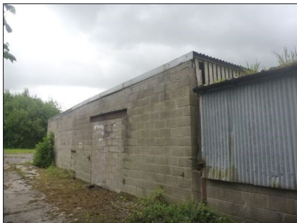
Photo 29: Building 4, section 4.1, north-eastern elevation
