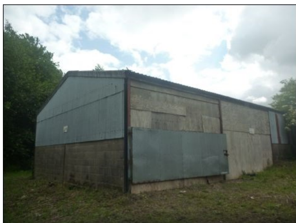
Photo 31: Building 4, section 4.5, south-western and north-western elevations
