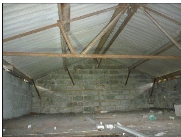
Photo 34: Building 4, section 4.2 roof void
