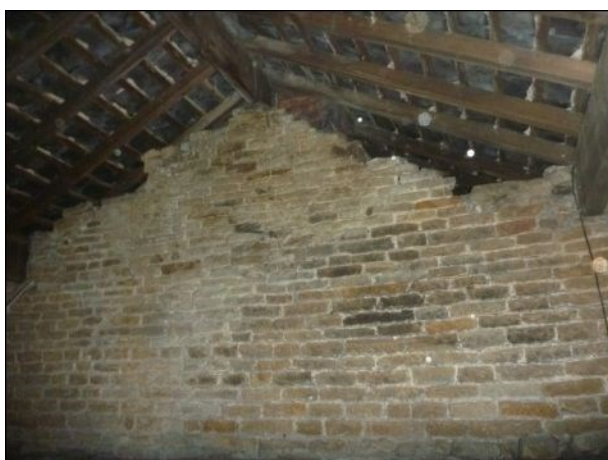
Photo 27: Building 3, roof void at south-eastern end of the building
