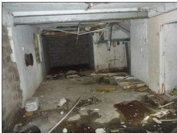
Photo 35: Building 4. Section 4.3 internal area
