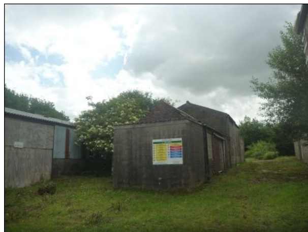
Photo 30: Building 4, sections 4.1, 4.2, 4.3 and 4.4, south-western and north-western elevations
