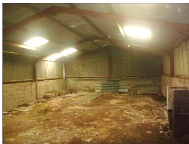
Photo 38: Building 4, section 4.5 internal area
