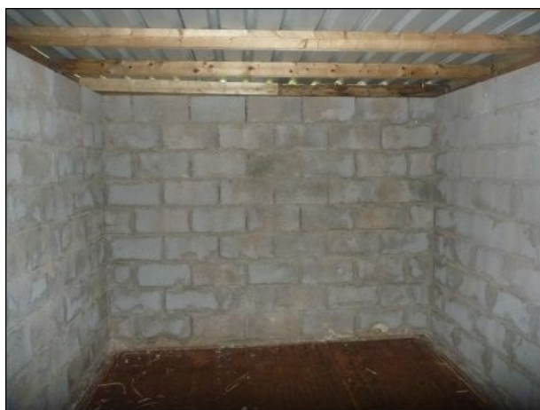
Photo 37: Building 4, section 4.4 internal area
