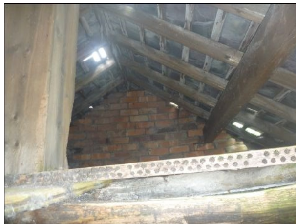
Photo 36: Building 4, section 4.3 roof void
