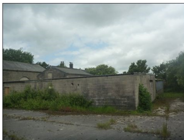
Photo 28: Building 4, section 4.1, south-eastern and north-eastern elevations
