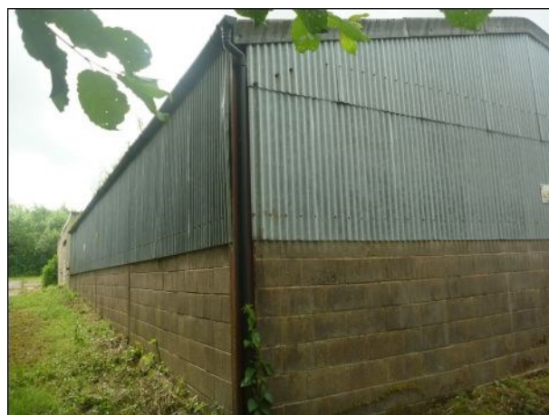
Photo 32: Building 4, section 4.5, north-eastern elevation
