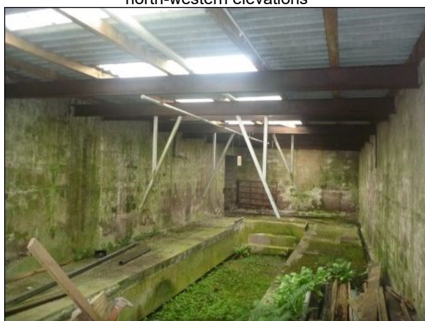
Photo 33: Building 4, section 4.1, internal area
