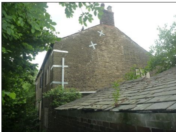
Photo 23: Building 3, south-eastern and south-western elevations
