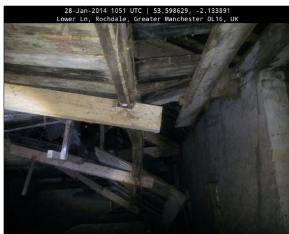
Photo 21: Building 2 internal area (photograph taken in 2014 and provided by the client)
