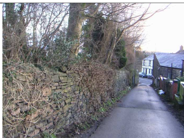
Photo 12: Western wall outside boundary line.
