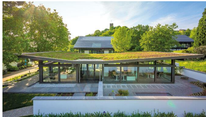
Sedum roof with metal fascia (zinc)
