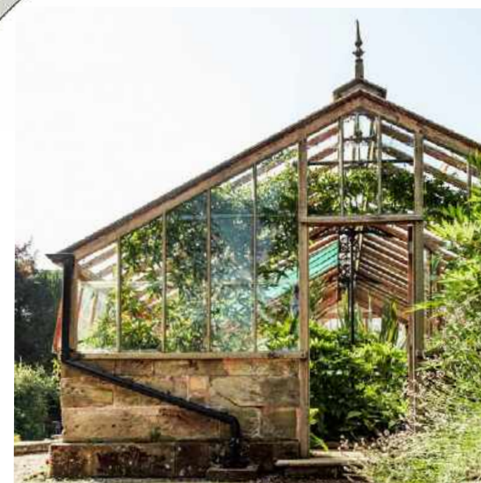
Communal greenhouse buildings in allotments and amenity spaces create shared facilities and encourage stewardship and group ownership
