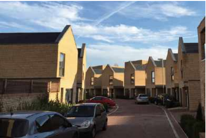
Example of insufficient space result in cars parked within the carriageway
