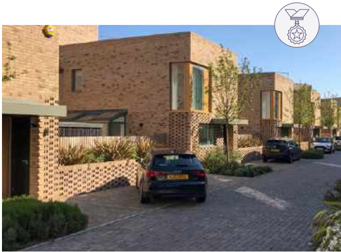
A subtle change in surface material demarcates parking punctuated by tree planting and soft landscaping
