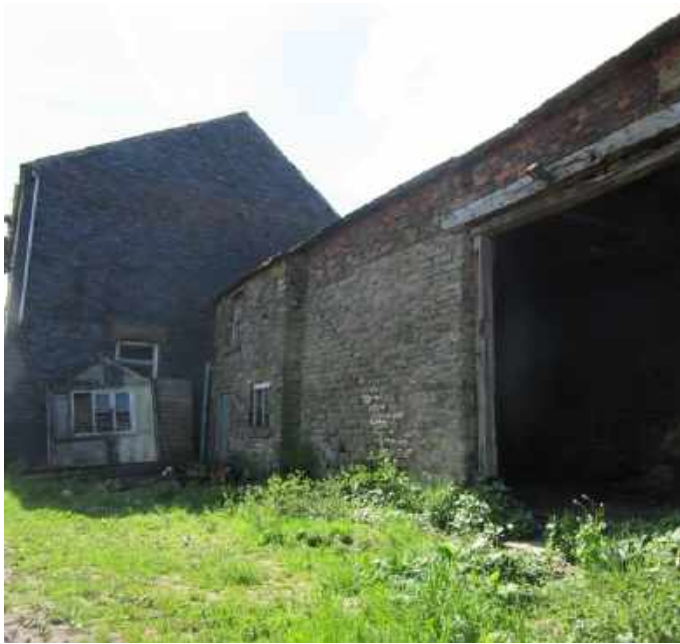
All buildings with confirmed bat roosts are proposed as retained as part of proposals, with additional bat boxes provided in key locations.
