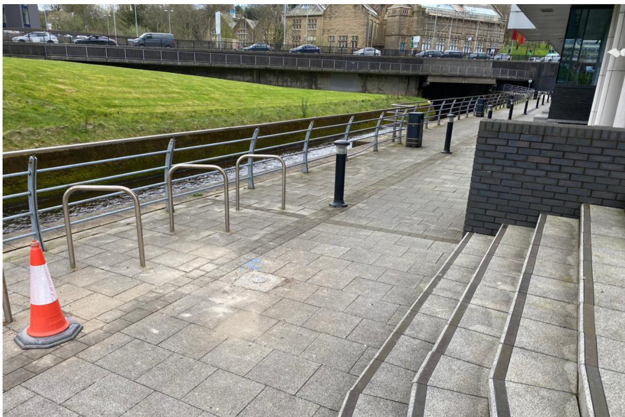
Photograph 6 – West aspect of the site next to the river and location of WS104.
