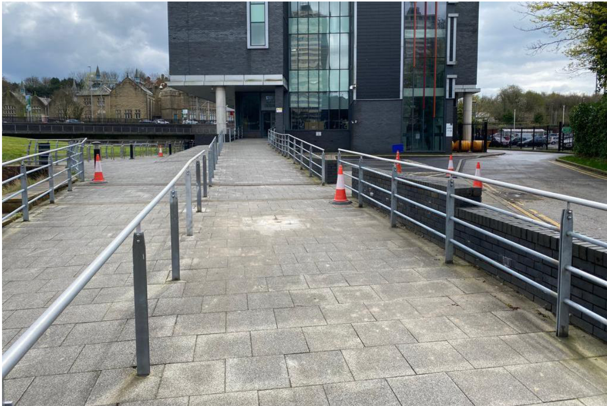
Photograph 3 – Walkway sloping upwards towards Rochdale Sixth Form Centre.
