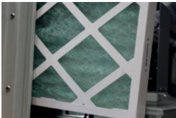
Figure 36 - UV-O 1000 Air Filter
