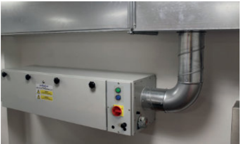
Figure 6 - UV-O 1000 Unit Installed
