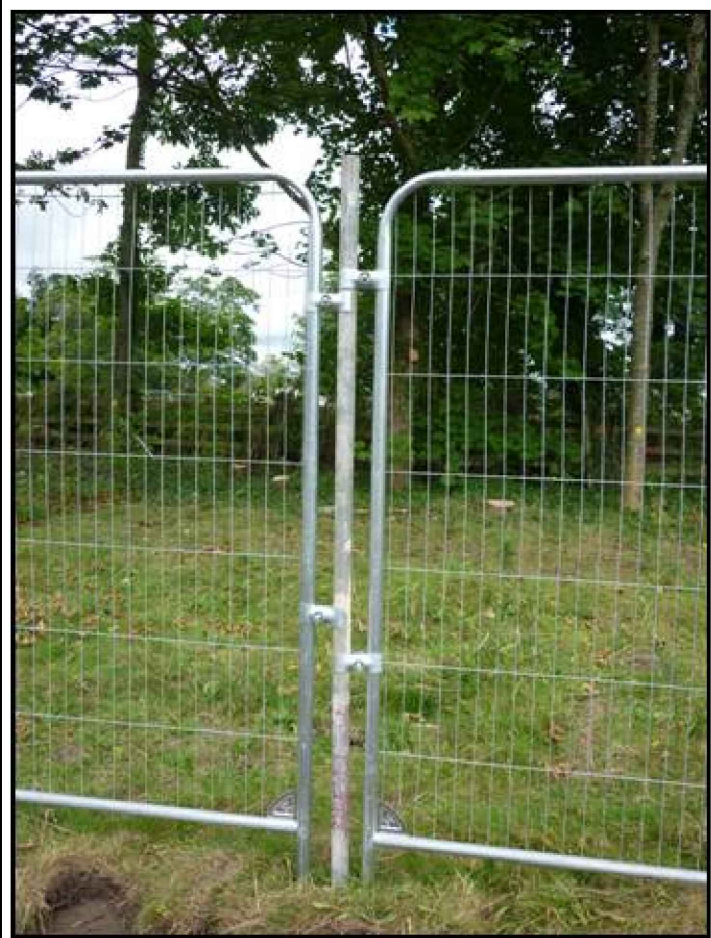
Tree Protective Fencing Specification
