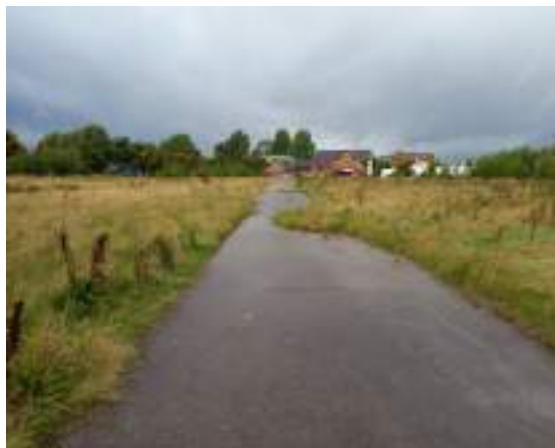
Photo 5— Hardstanding section running east/west.
