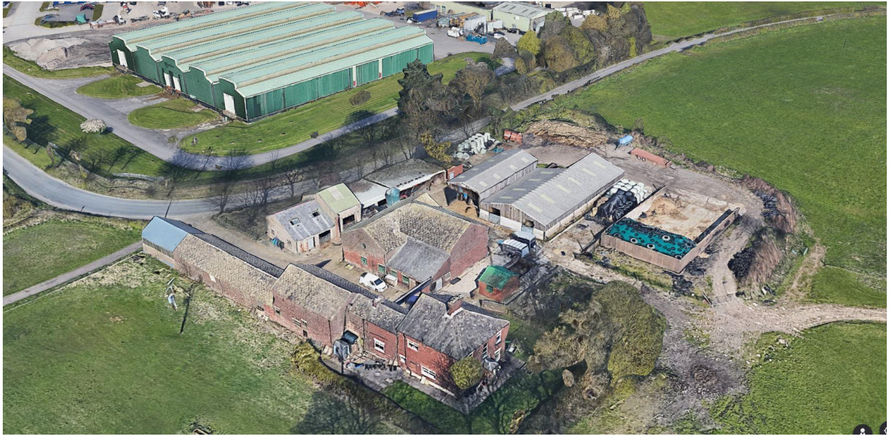
Figure 4-1. 3D model showing Broom Hill Farm. Source: Google Earth View, July 2019.
